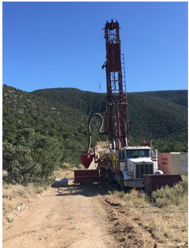
Investigative operations at the Burn Site Groundwater Area of Concern.
