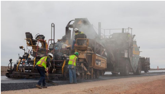
Workers lay asphalt, completing the new WIPP bypass road.
