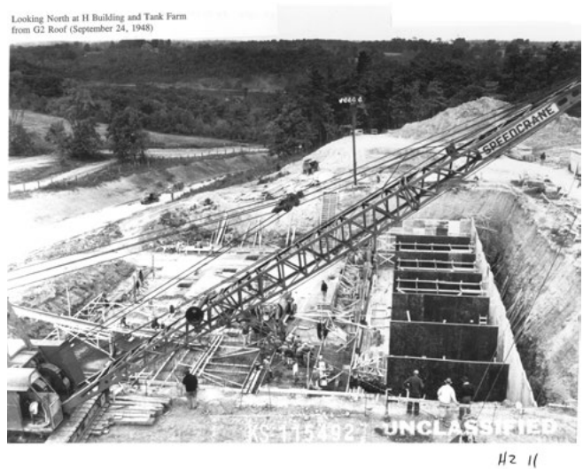
Building H2 in 1948, showing construction of tank vaults.
