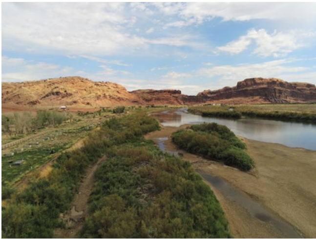
A side channel of the Colorado River adjacent to the Moab Site was mostly dry in July. In addition to extraction wells that remove contaminants from groundwater underlying the site, the concrete vaults (seen here on the left) house injection wells that create a hydraulic barrier to help prevent constituents from entering the river.
