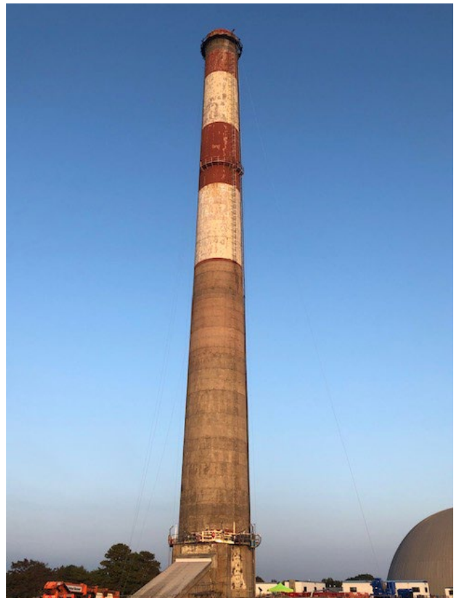
Western facing half of stack abatement progress as of October.
