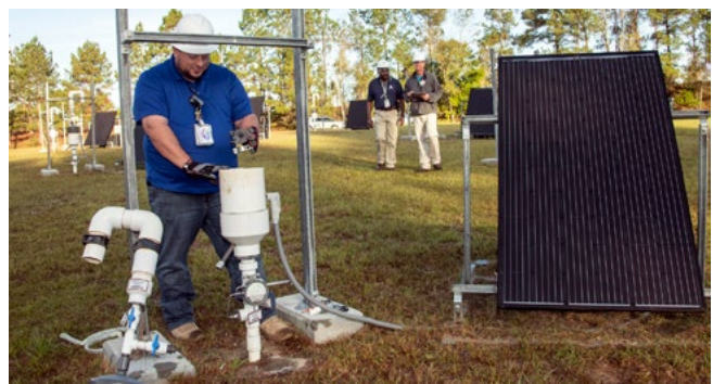
SRS engineers check components of a MicroBlower unit and inspect the solar panels that power the unit in the M-Area Settling Basin.
