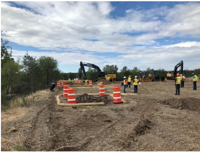
Workers dig a trench on former LANL along DP Road.
