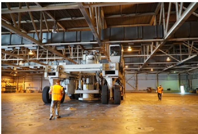
A Shielded Canister Transporter is used to double-stack canisters in Glass Waste Storage Building 1.
