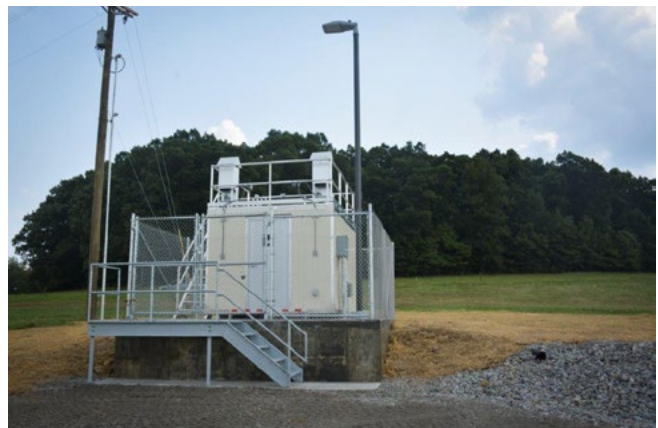
One of five co-located air monitors at the site that will allow for parallel analysis of sampling data with OEPA during site demolition.
