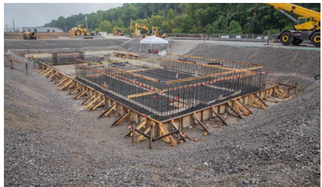
Workers poured the foundation for the Mercury Treatment Facility this year.
