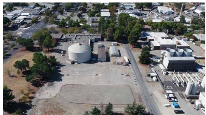
Looking west across the Building 280 area in October.
