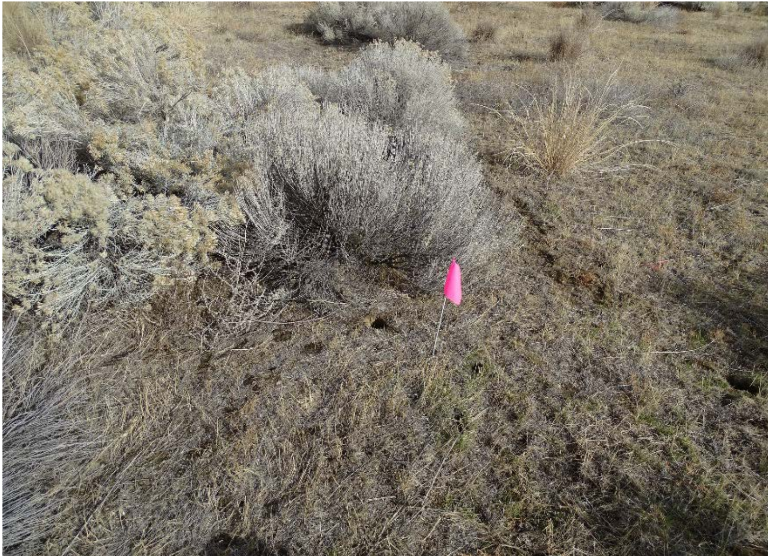
Location 6 - Subsidence Area near Opening to the H-12-L Battery B Nike Underground Missile Storage Structure
