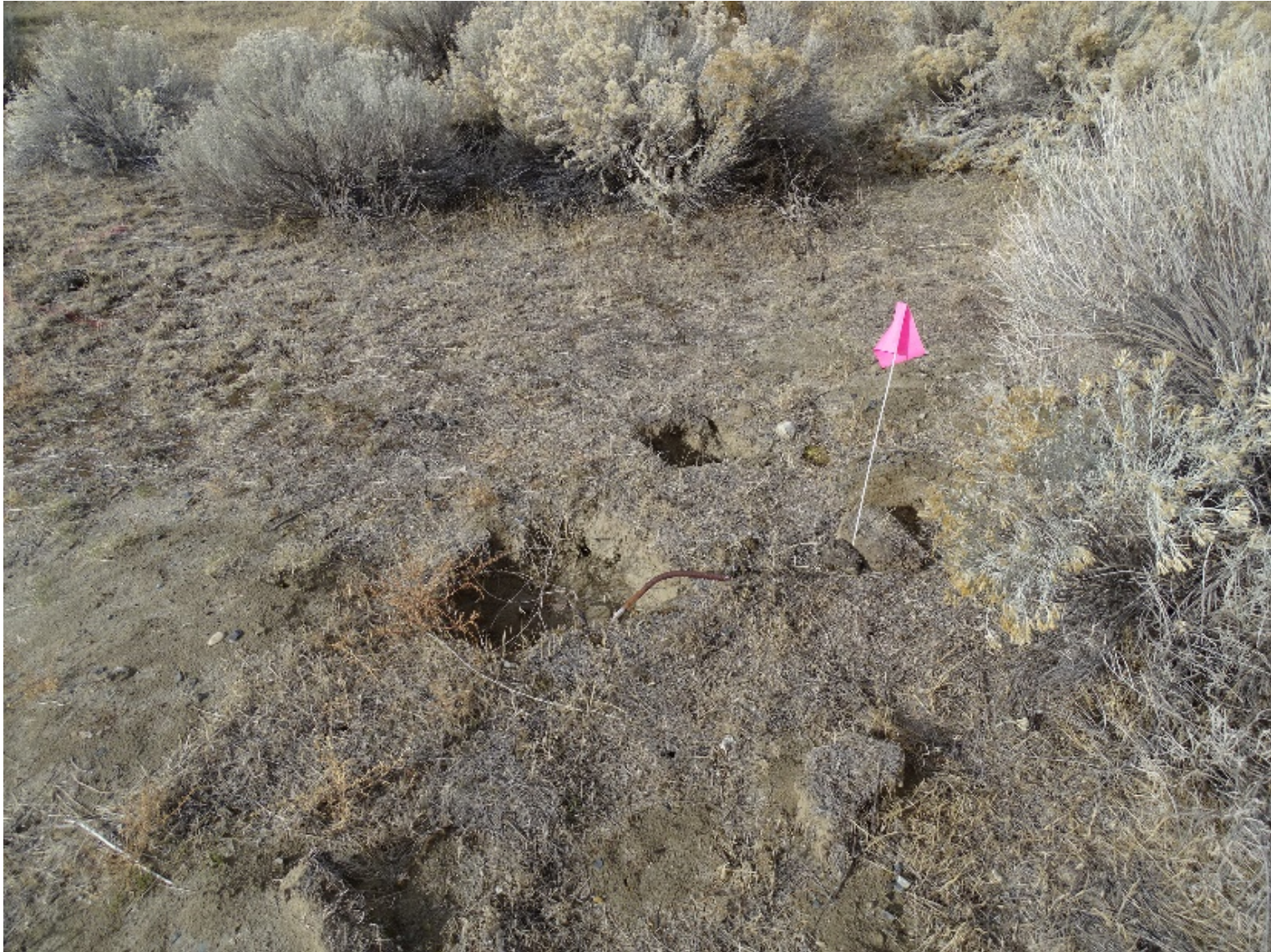
Location 2 - Sinkholes Adjacent to Filled Stairwell Entrance to the H-12-L Battery B Nike Underground Missile Storage Structure
