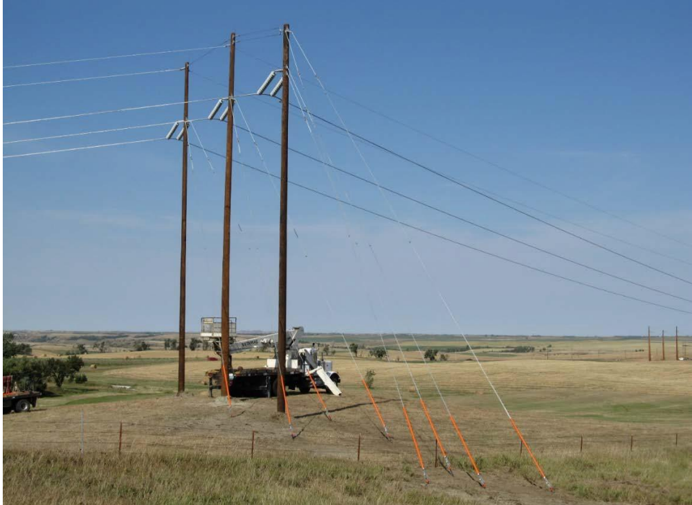
Photo 1: Guy wire installation
