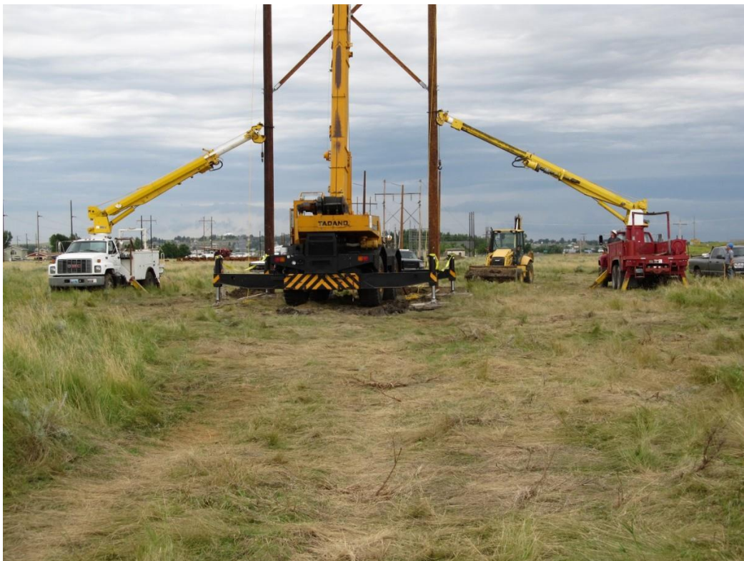
Photo 6: Equipment and disturbance during installation of structures.
