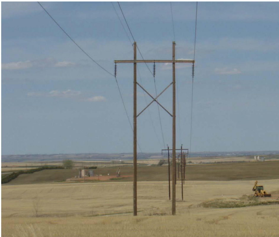
Photo 4: The structure in the foreground is an example of the structure design that WAPA is proposing to install. The structures in the background are the original structures, which WAPA is proposing to replace (up to 30 deteriorated structures).
