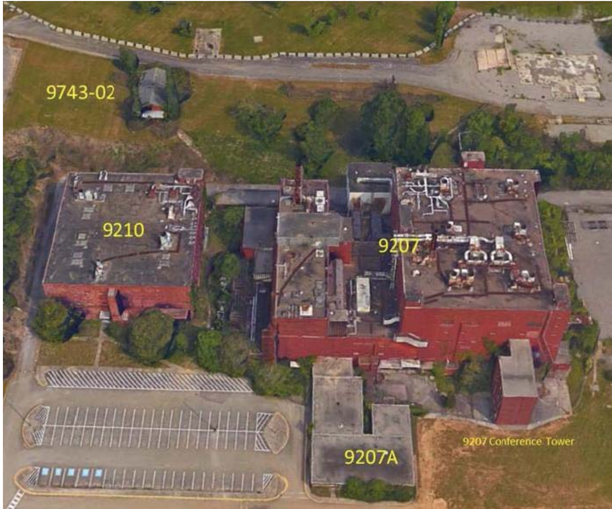
Figure 2-2. Existing Biology Complex Site Facilities
