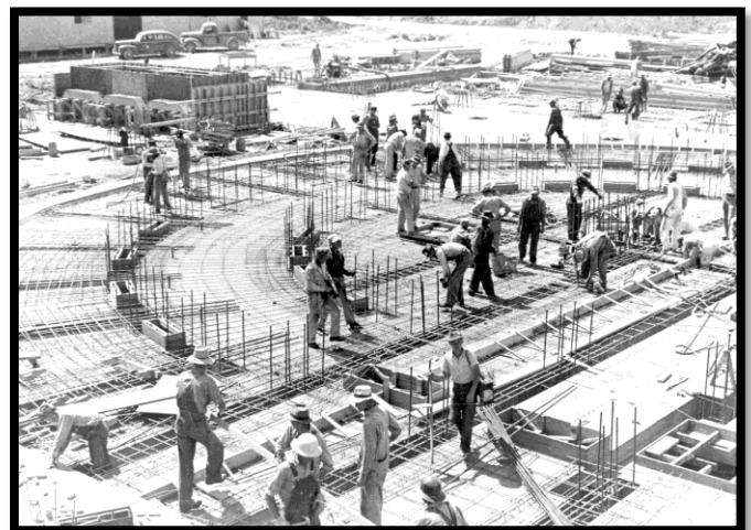
Historical photo of an alpha racetrack under construction, Y-12, Oak Ridge. Photo taken 1943.
