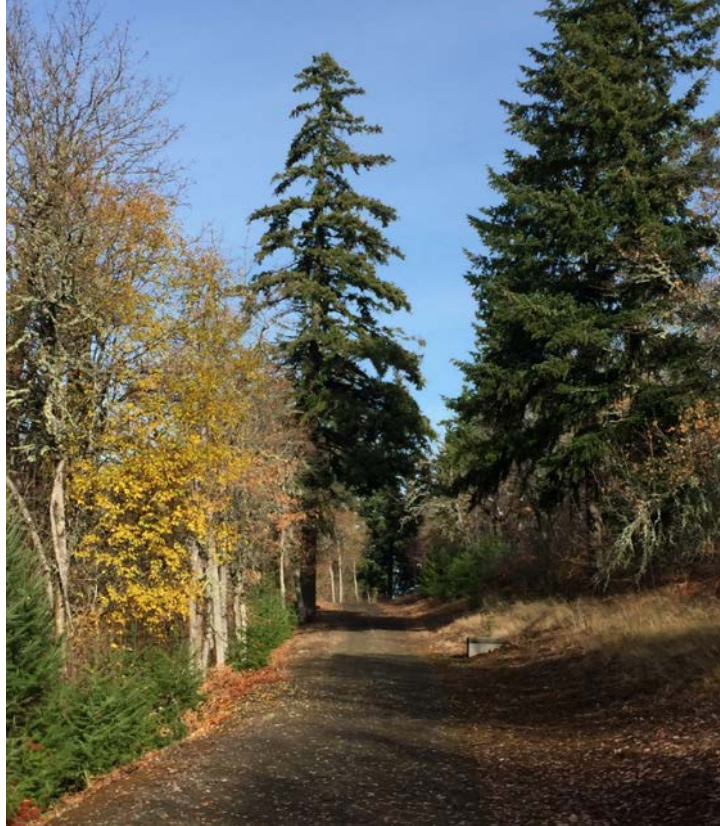
Figure 6-1. A section of the Central Lateral Pipeline 9 years after construction.
