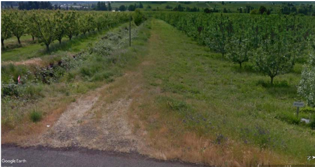
Figure 6-2. Vegetation along a buried District lateral pipeline 5 years after construction.
