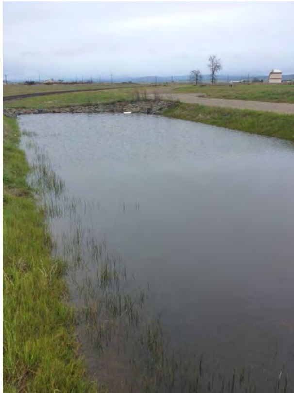
Photo 23. Settling basin (Beale AFB) [-121.417659, 39.101091] – Facing South
