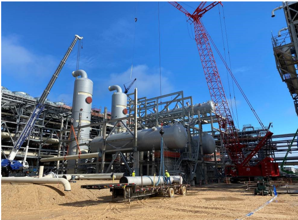
Progress at Propane Refrigeration area
