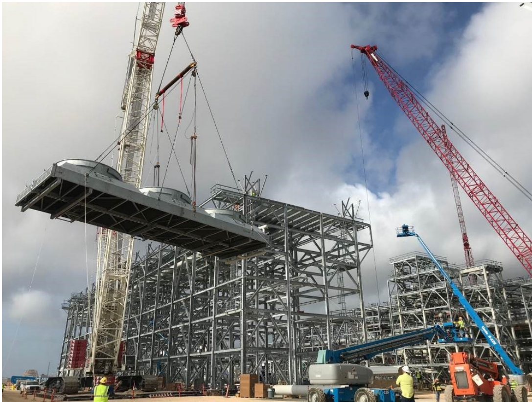
First Propane Refrigeration Condenser (Fin Fan) being set at Train 6
