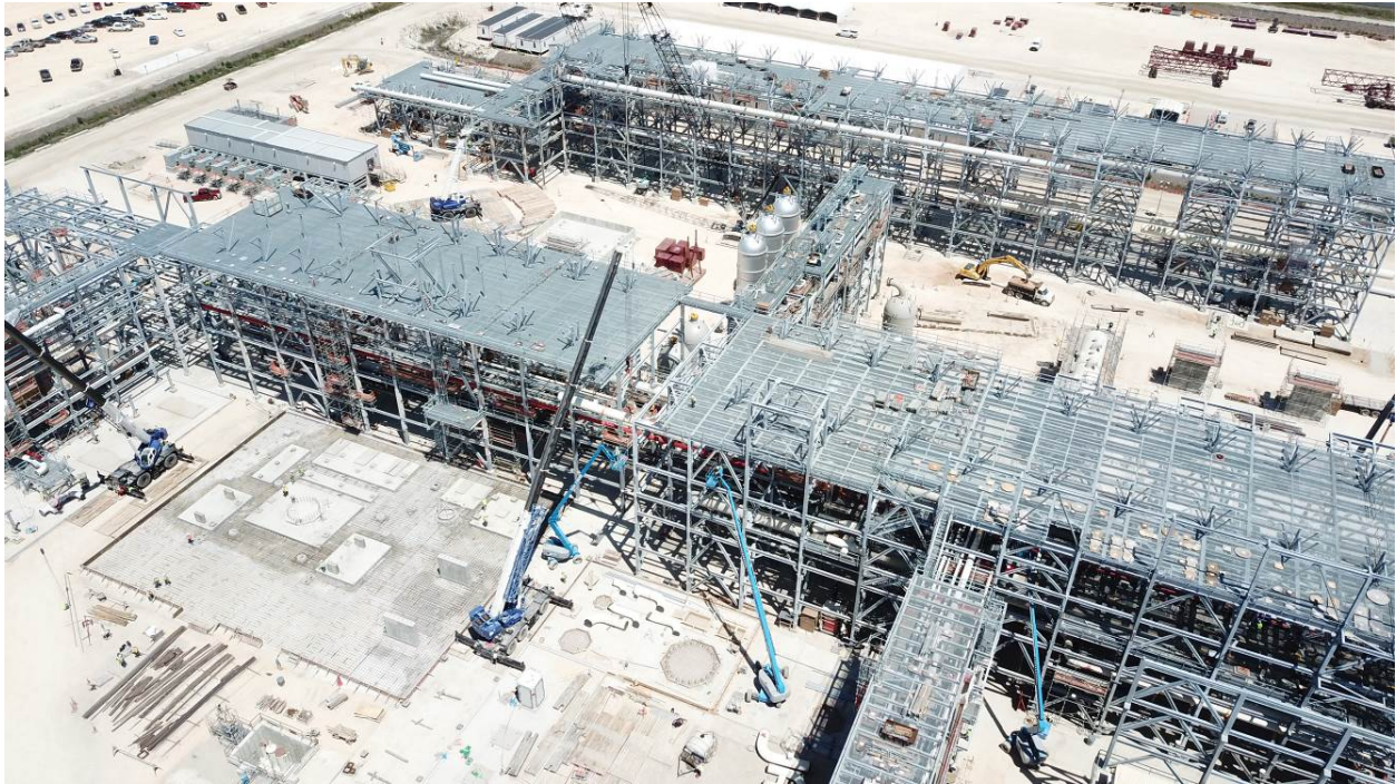
Steel and pipe progress in Train 6
