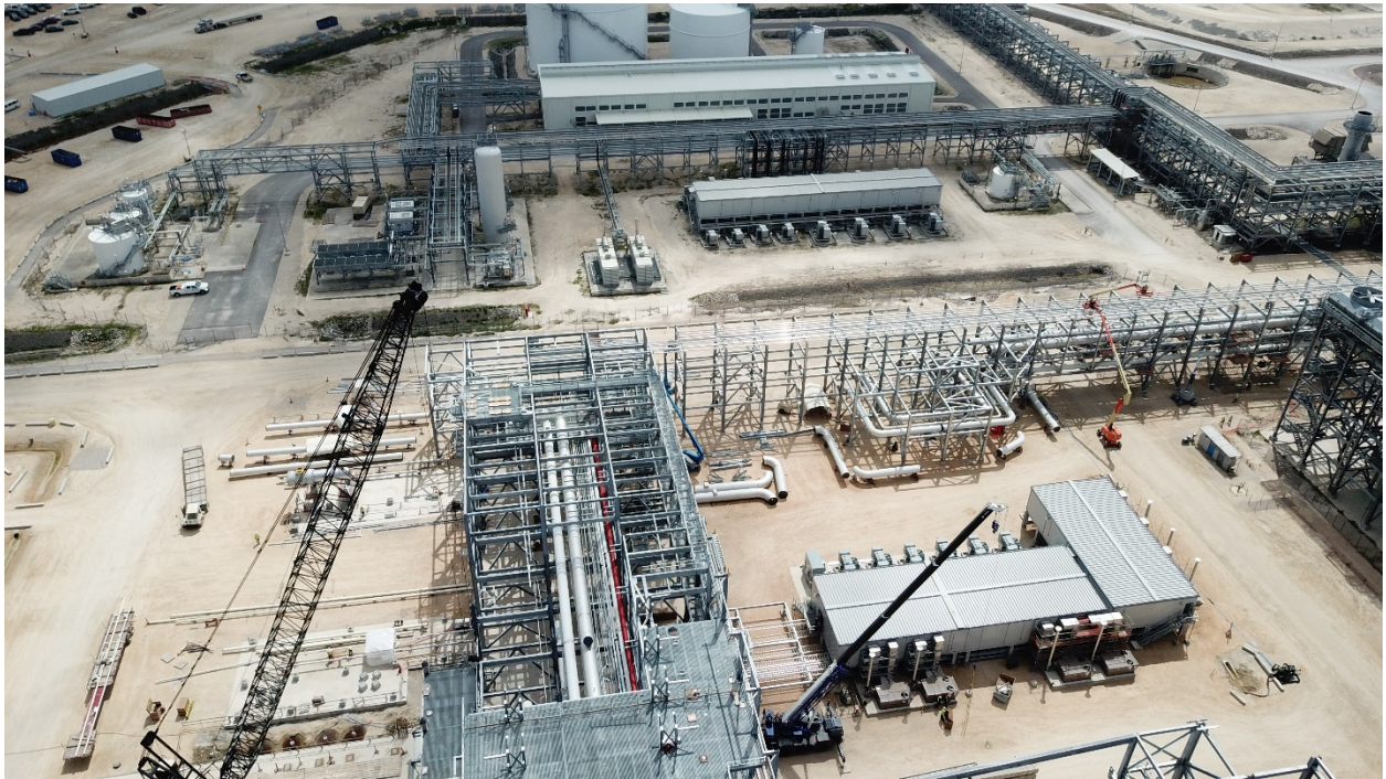
Steel and pipe progress at south end of Train 6
