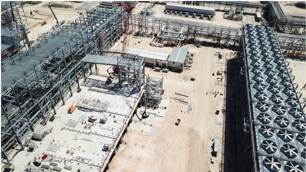
Progress at south end of Train 6
