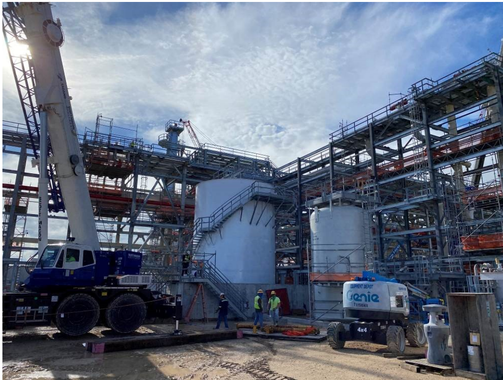
Amine Surge Tank Completed
