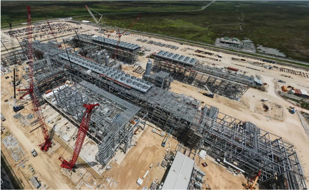
Progress at Train 6 facing East
