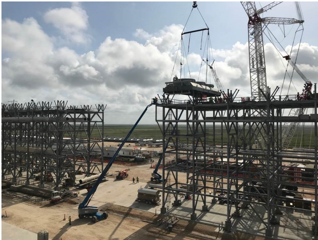
First Propane Refrigeration Condenser (Fin Fan) set at Propane Condenser Rack
