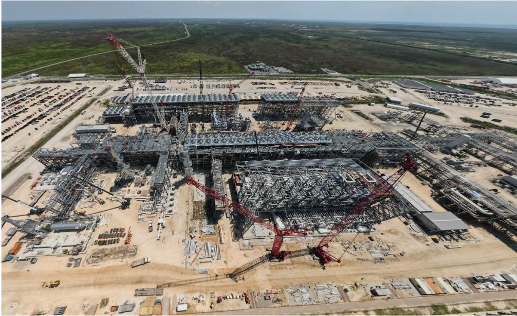
Progress at Train 6 facing East
