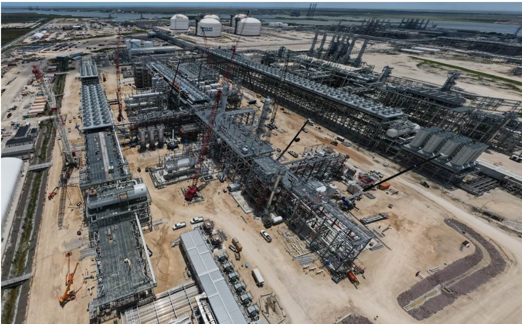
Progress at Train 6 facing South
