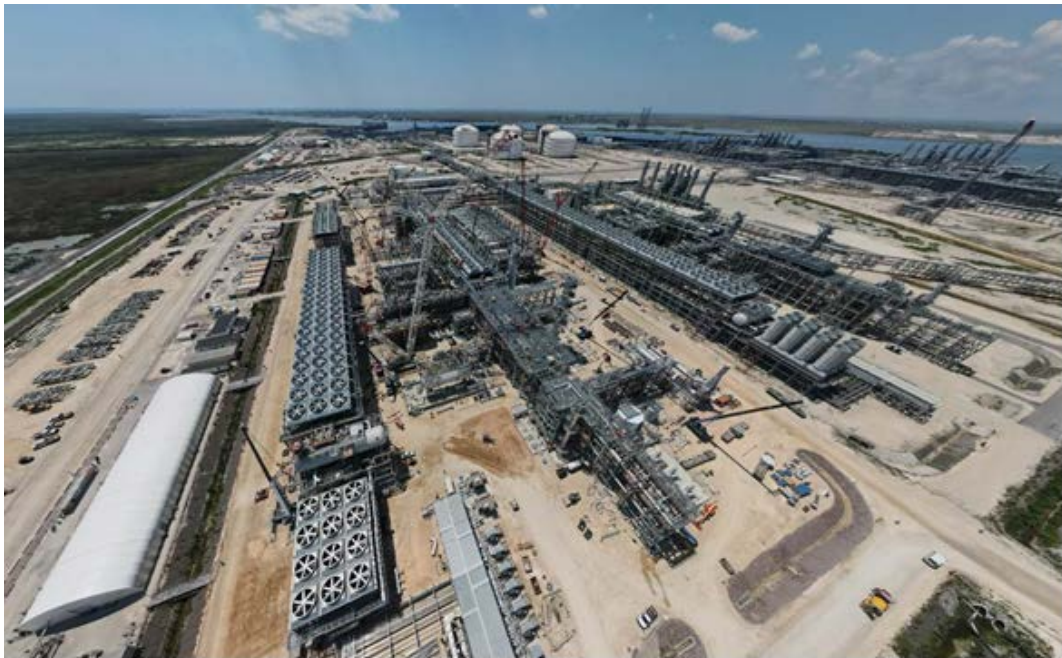
Progress at Train 6 facing South
