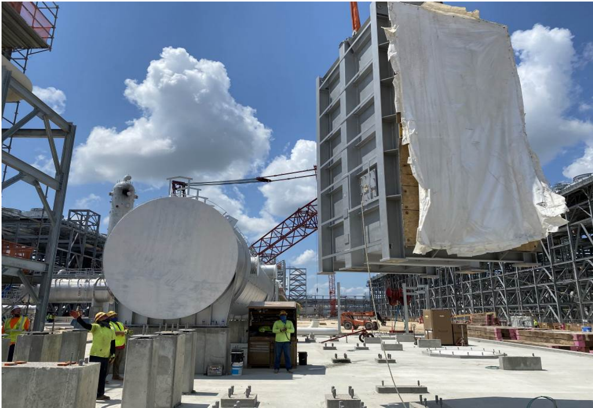
Thermal Oxidizer Pre-Heater being set
