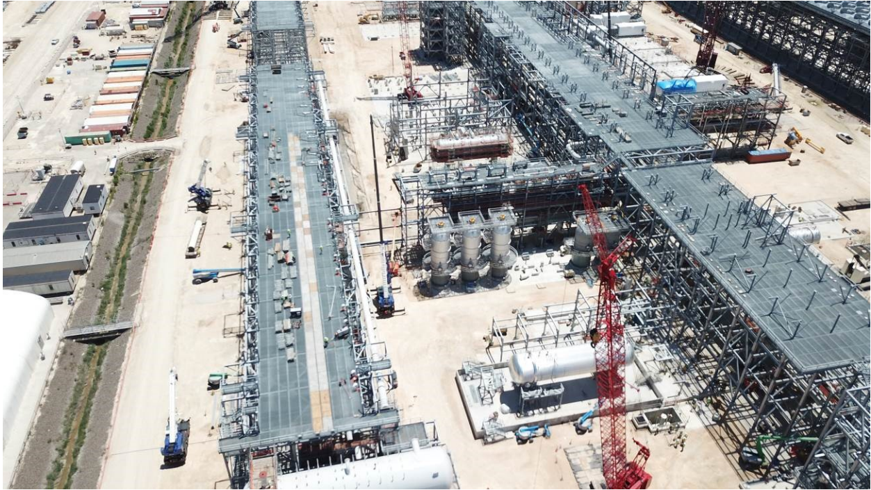
Progress as seen from North end of Train 6
