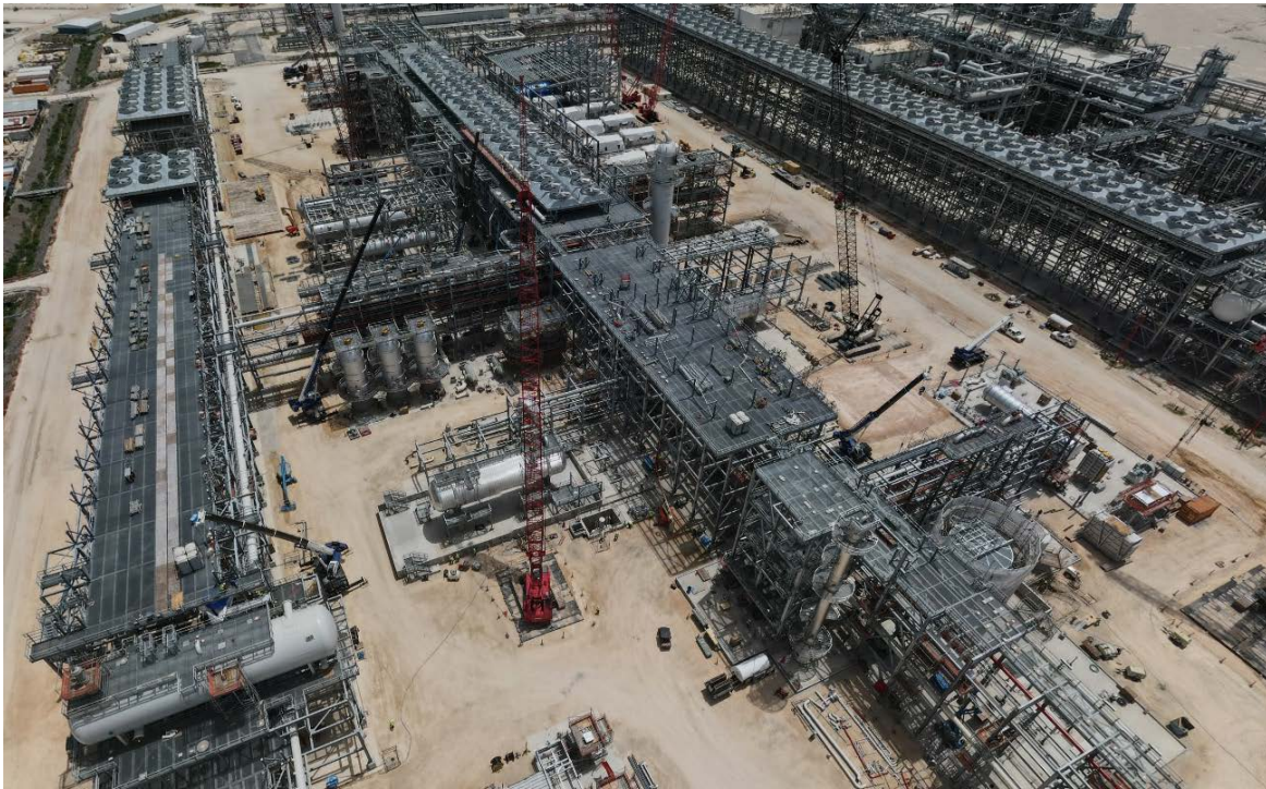
Progress as seen from North end of Train 6
