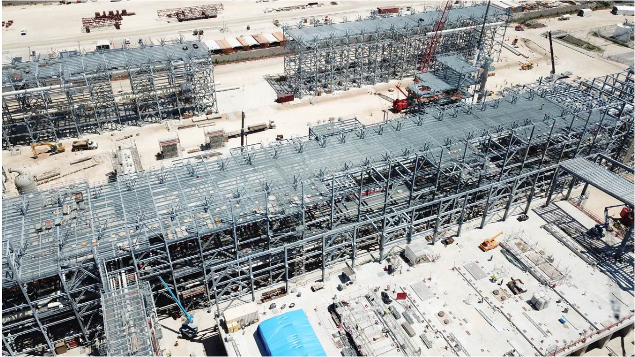
Progress at Train 6
