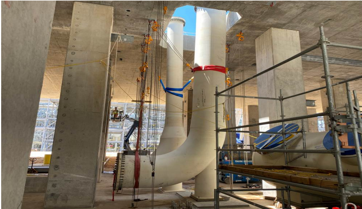
Final Hockey-stick pipe in Propane Section of Compressor Area
