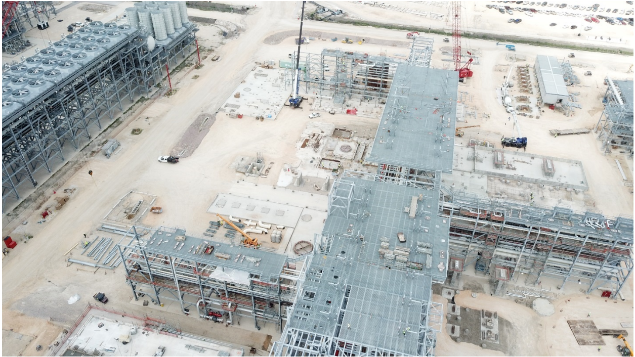
Progress at northeast side of Train 6
