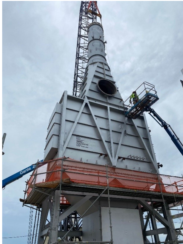
Progress at Thermal Oxidizer
