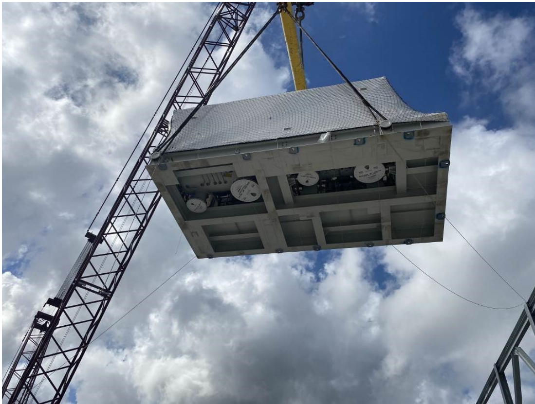
First Compressor being set at Train 6
