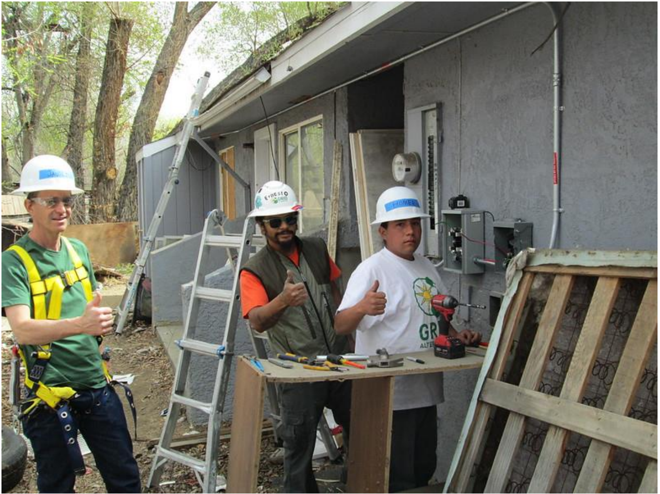
Inverter wiring training with Tribal members
