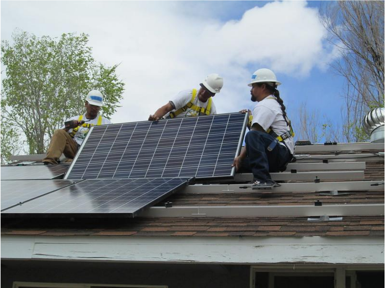
Roof training with Tribal trainees
