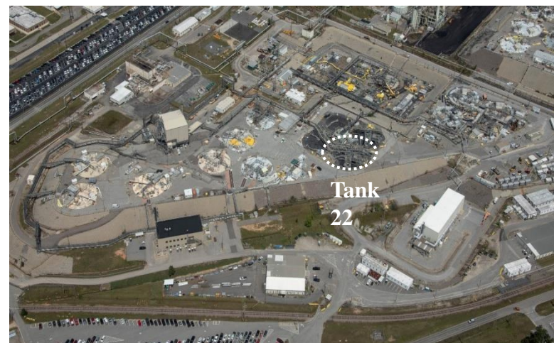
Aerial view of Tank 22 and H Tank Farm
