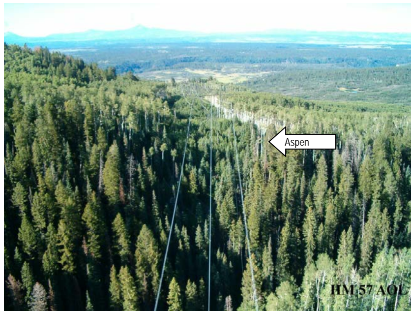
Photo 2-4. Incompatible conifer and aspen vegetation that would require initial treatment to establish a low-growth condition, which WAPA would then maintain. In the middle of the photo, note how the aspen in the ROW have vigorously re-grown after numerous treatments.
