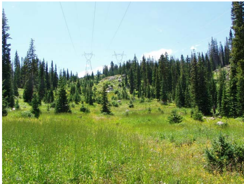
Photo 2-12. These two parallel lines have different authorizations for vegetation maintenance. The line on the left is in a desirable condition, but WAPA will monitor it and treat as needed. The line on the right is not in a desirable condition; WAPA would schedule it for initial treatment and then maintain it in a condition similar to the line on the left.
