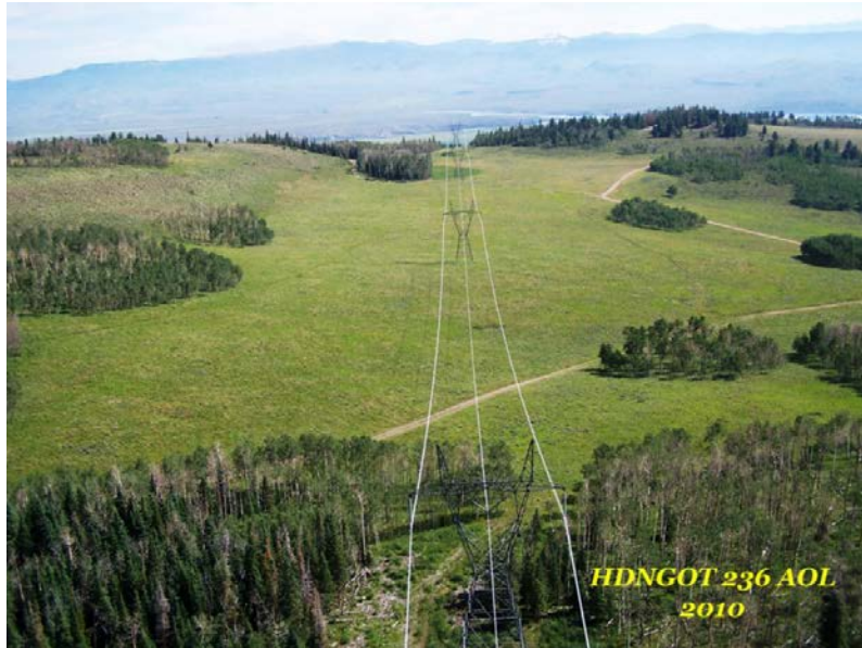
Photo 2-1. ROW with natural, low-growing vegetation outside the aspen stands that is compatible with the transmission line.
