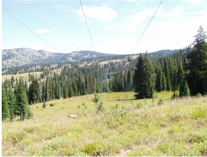
Photo 2-15. Although this ROW is generally acceptable, the two larger trees under the transmission line are due for treatment to ensure they do not present a hazard to the line.
