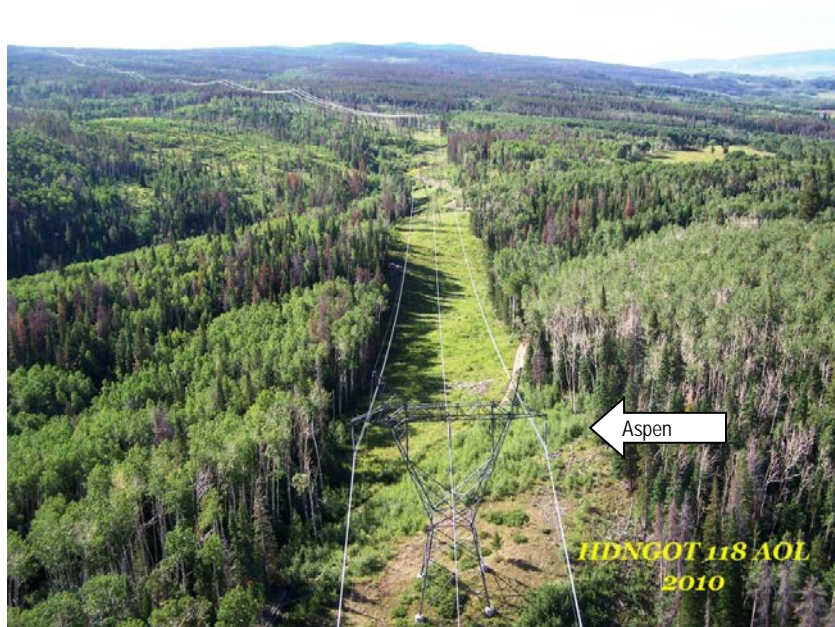
Photo 2-7. The ROW was cut when the line was constructed and has been maintained in a desirable condition. Note that aspen and lodgepole pine are the predominant species, with rapid aspen regeneration occurring immediately behind the first transmission line structure. WAPA would monitor the ROW and treat it as needed to maintain this condition.
