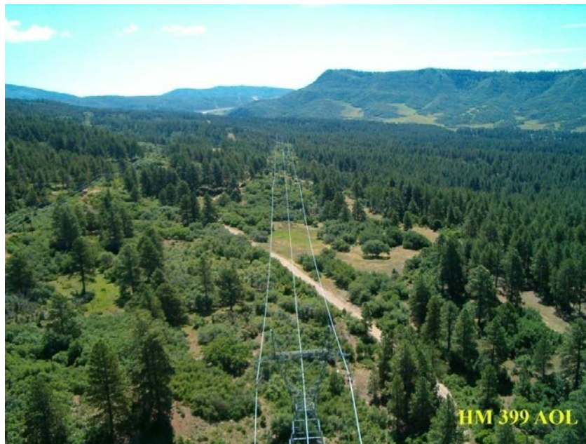
Photo 2-16. WAPA would monitor potential fuel loading under the lines and near the structures, and schedule treatment as needed.
