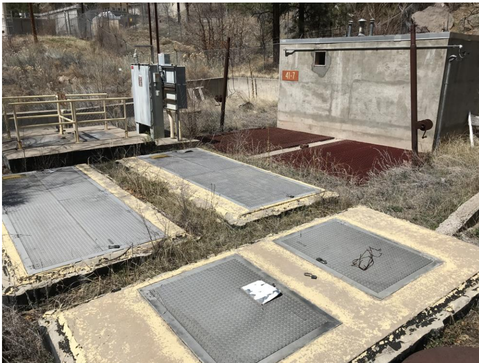
Photo 2. View of former waste water treatment facility (41-0007).
