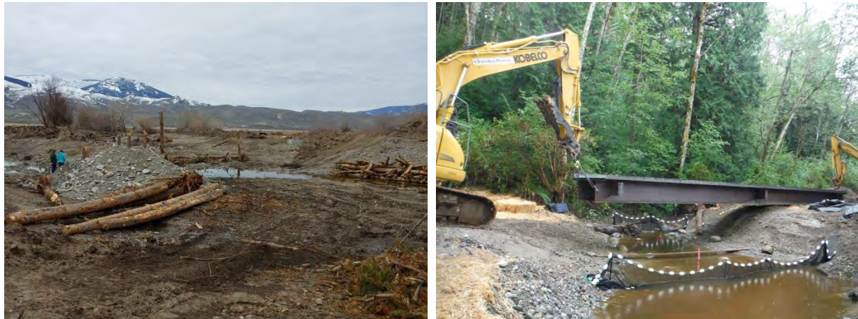
Figure 5 Range of construction activity impacts from restoration projects
