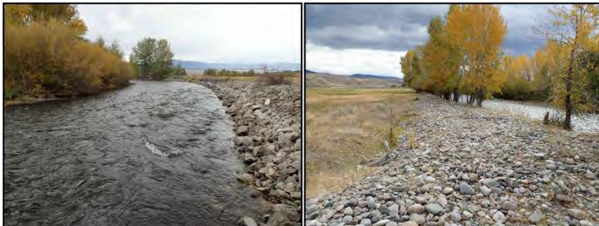
Figure 7 The Lemhi River disconnected from its floodplain at Eagle Valley Ranch
