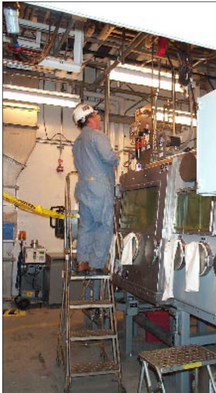
PuSPS under construction
