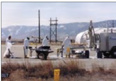
Workers conduct sampling on the 903 Pad
