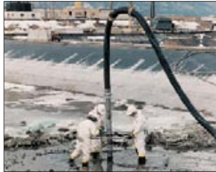
Workers remove sludge from the Solar Evaporation Ponds
