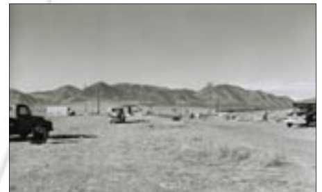
Construction begins on the west gate
