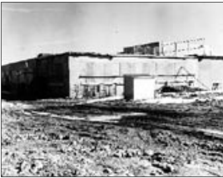
Building 444 under construction in 1951
