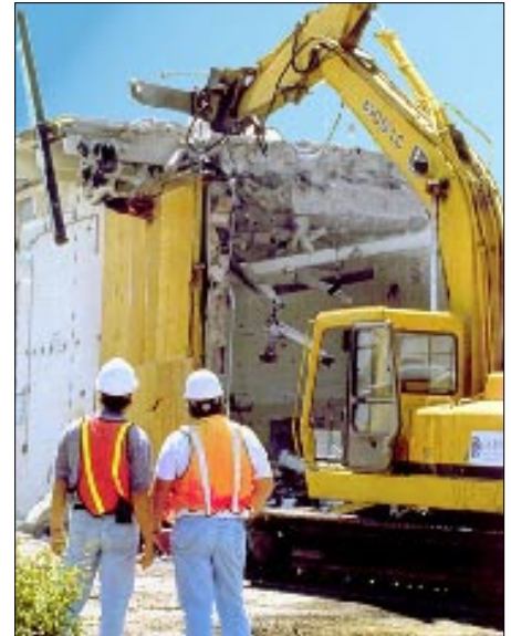
Building 889, the first radioactively contaminated structure to be demolished
