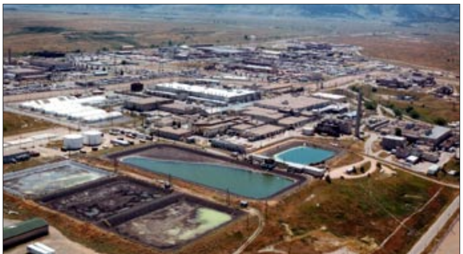
Solar Evaporation Ponds
