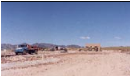
Construction of the East Access Road
