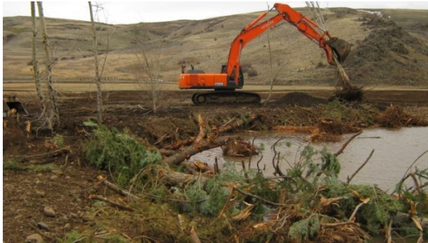
Figure 4. 300 series Track-mounted excavator
