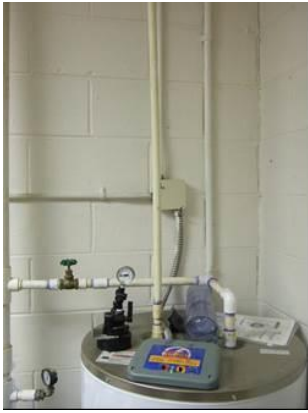
Insulate hot water lines
