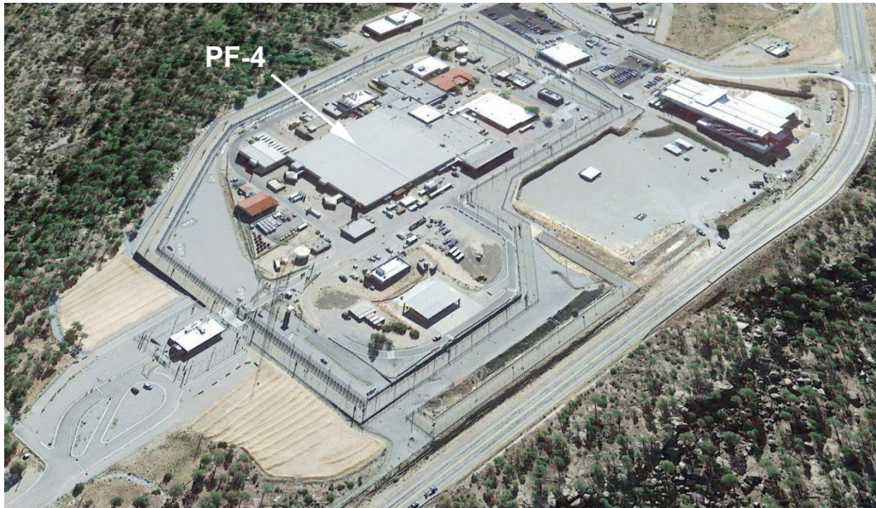
Figure 2-2. The Plutonium Facility Complex at TA-55 with (PF-4) identified.
