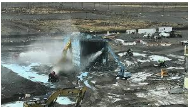
Photo 1. Demolition of the Plutonium Finishing Plant
