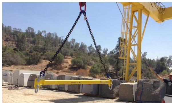
Photo 4. Example of a spreader bar used for hoisting and rigging
