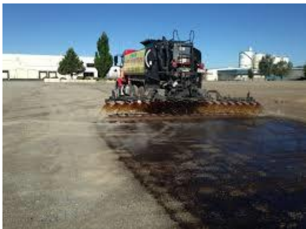
Photo 3. Application of dust palliatives for dust suppression
