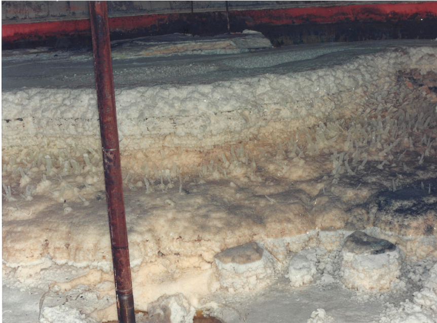
FIGURE 3.2 Interior of a Hanford tank showing layers of saltcake and sludge. The tank wall is in the far background. The pumpable liquids have been removed from the tank. SOURCE: Department of Energy.
