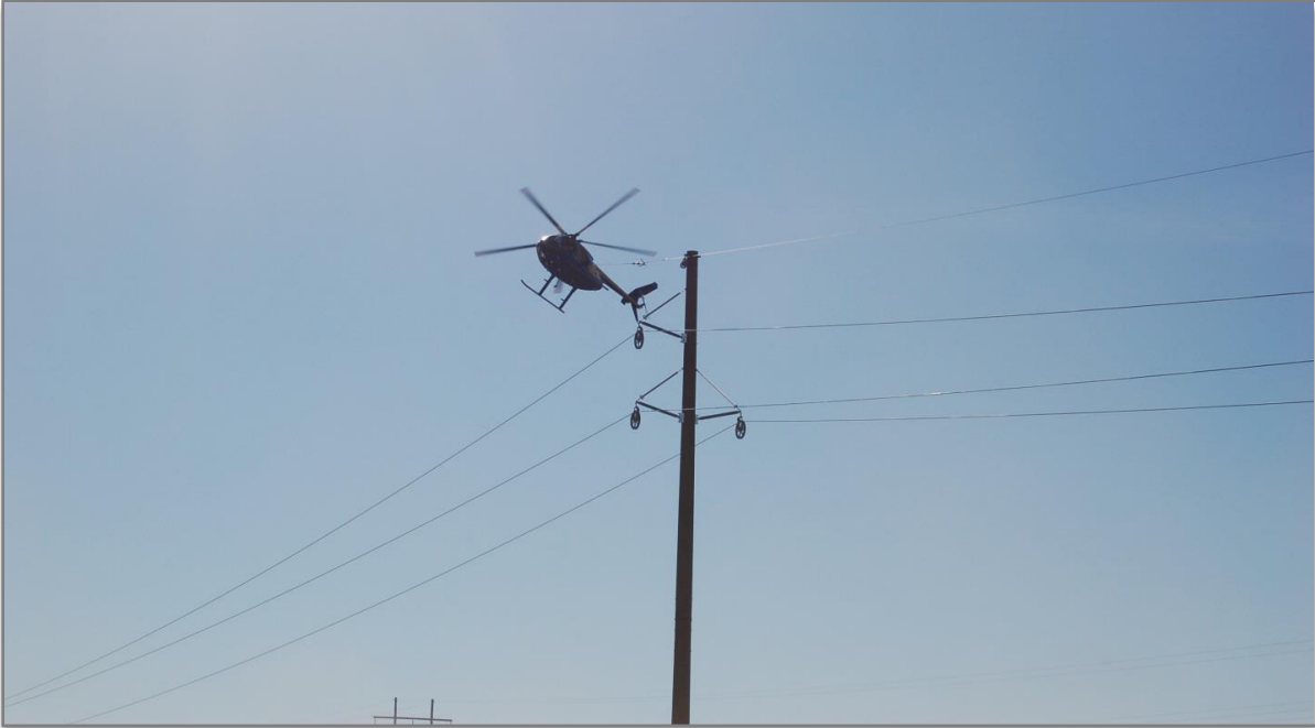
FIGURE 3-3. HELICOPTER ASSISTED INSTALLATION SHIELD WIRE TRANSFER (CENTURYLINK AND PNM 2019)
