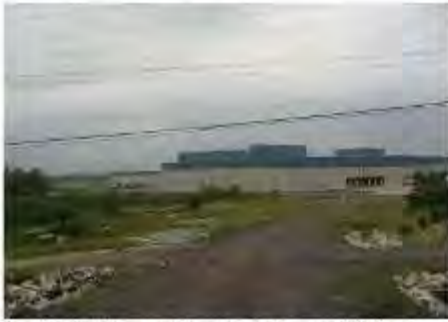
Location 1 looking northeast toward nearest building.
