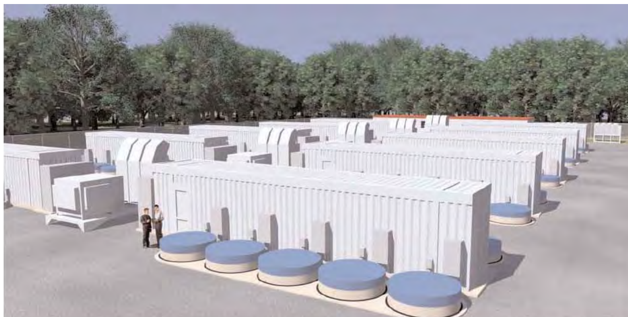
Figure 2-4. Array of 1-megawatt frequency regulation pods.
