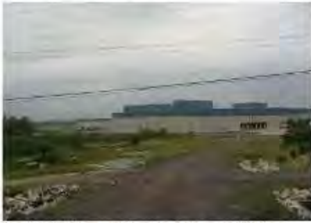
Location 1 looking northeast toward nearest building.
