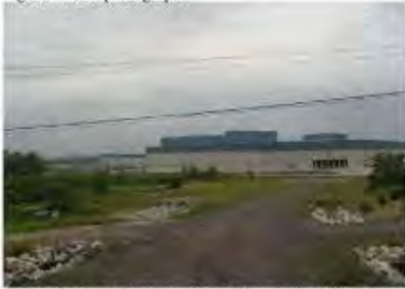
Location 1 looking northeast toward nearest building.
