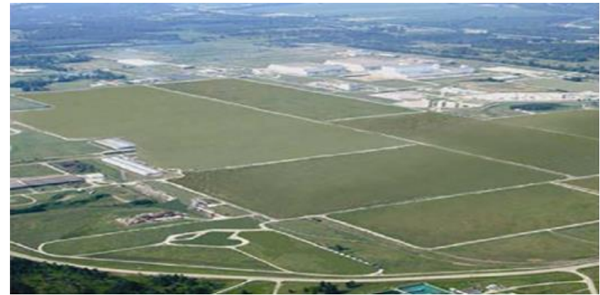
Future vision of central plant after D&D is complete
