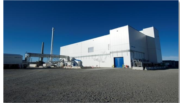
Integrated Waste Treatment Unit
