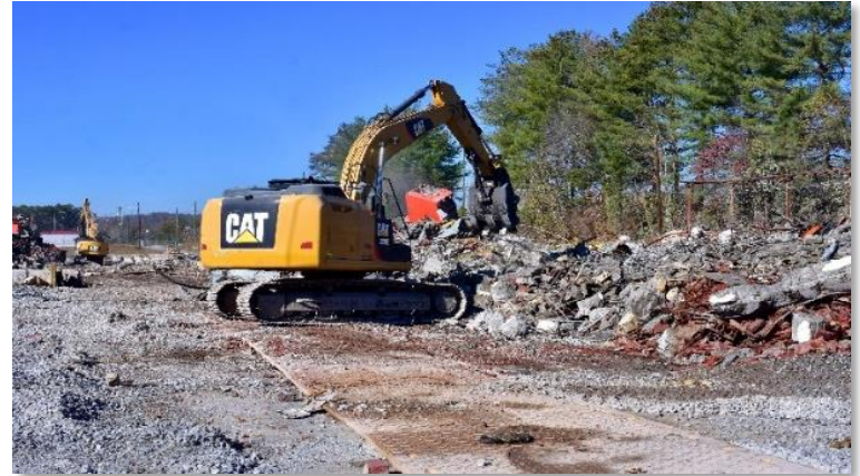
Demolition of East Tennessee Technology Park facilities
