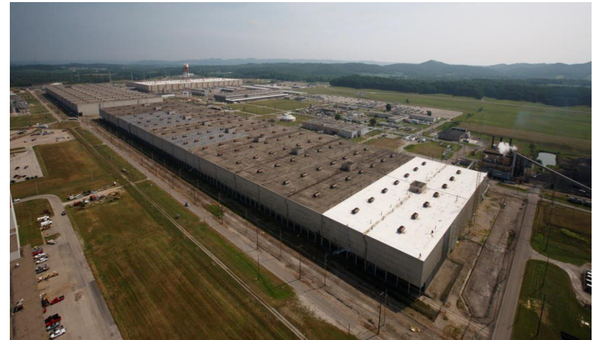
Process Building X-326 at Portsmouth
