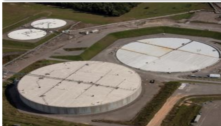
Saltstone Disposal Unit 6/7 at the Savannah River Site
