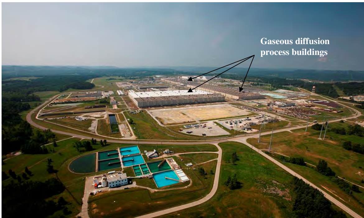
Figure 1.1 The Portsmouth Gaseous Diffusion Plant.
