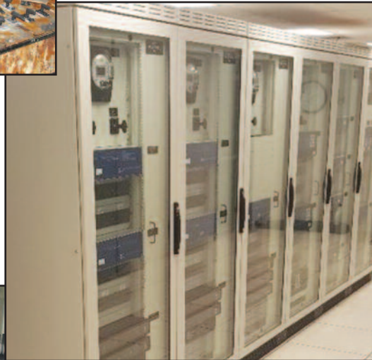
New protective relay and metering cabinets (above) and sootless generator floor.
