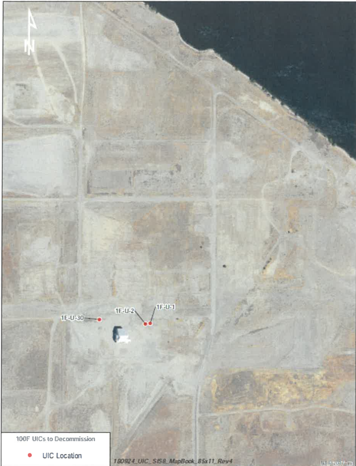
Figure 4. UIC Wells 1F-U-1, 1F-U-2, and 1F-U-30 Aerial Photograph in 100-F Area
