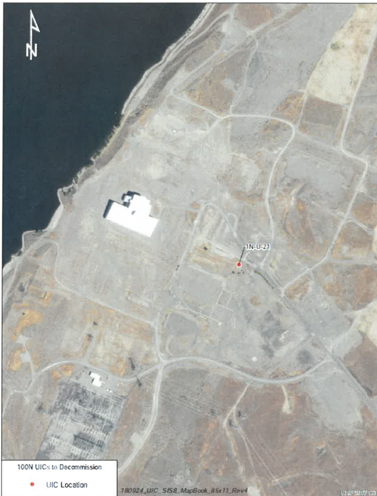
Figure 6. UIC Well 1N-U-21 Aerial Photograph in 100-N Area
