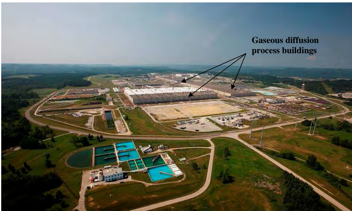
Figure 1.1 The Portsmouth Gaseous Diffusion Plant – 2011.
