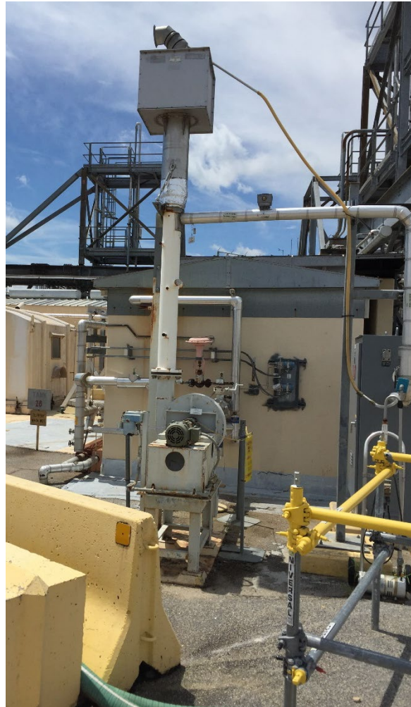
Figure 1. Modified Ventilation Exhaust Stack
