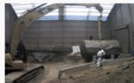
2011: Removal of Tank W1A at ORNL
