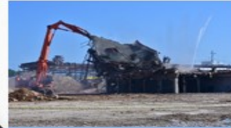
2016: Demolition of K-27 Completed
