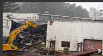
2019: Demolition of K-1037 Completed
