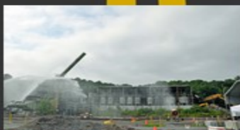
2018: Demolition of TSCA Incinerator Completed
