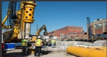
2017: Initiated Construction of Outfall 200
