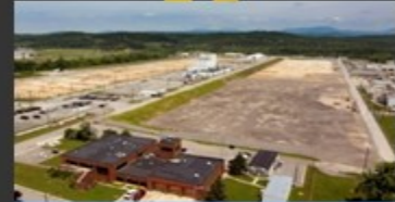
2014: Demolition of K-25 Completed
