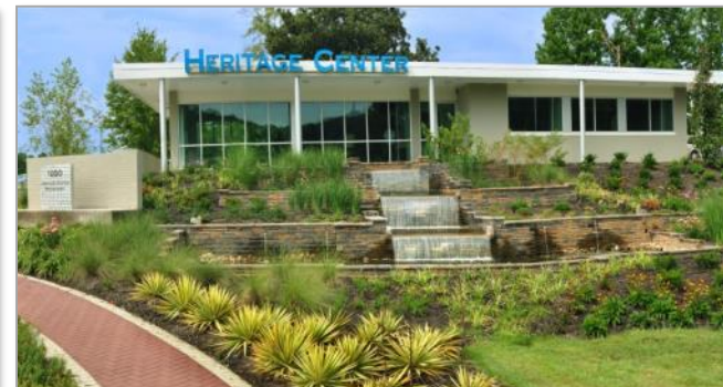
Heritage Center Industrial Park at ETTP
