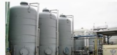
2019: Completed Installation of GAC Columns at Building 3608
