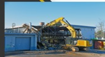
2019: Demolition of K-1414 Completed
