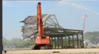
2015: Demolition of K-31 Completed
