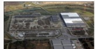
2011: Building K-33 at ETPP Demolished
