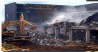
2006: Building K-29 at ETPP Demolished
