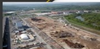
2010: Building K-25 West Wing Demolished
