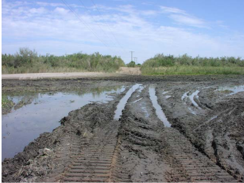
Figure 3.4-3. Transmission Line Crossing of Gila River.
