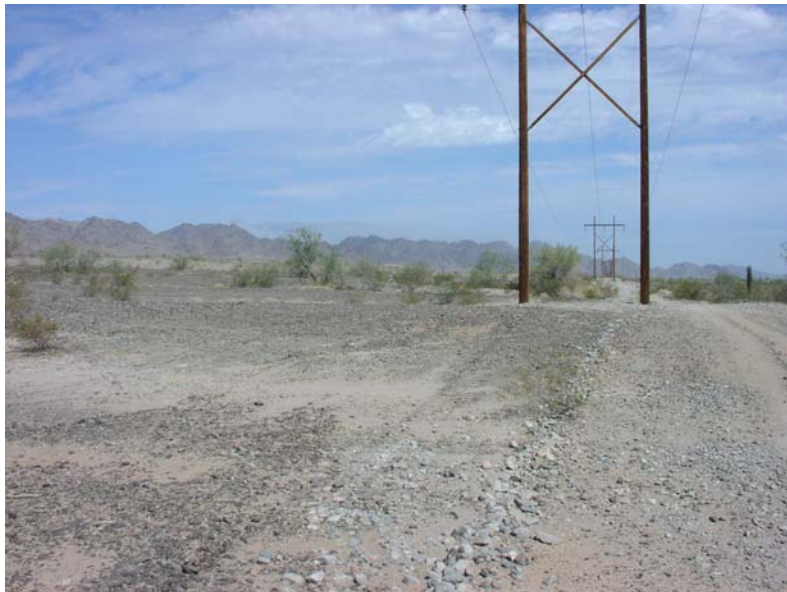
Figure 3.4-2. Typical Desert Pavement on Transmission Line Route.
