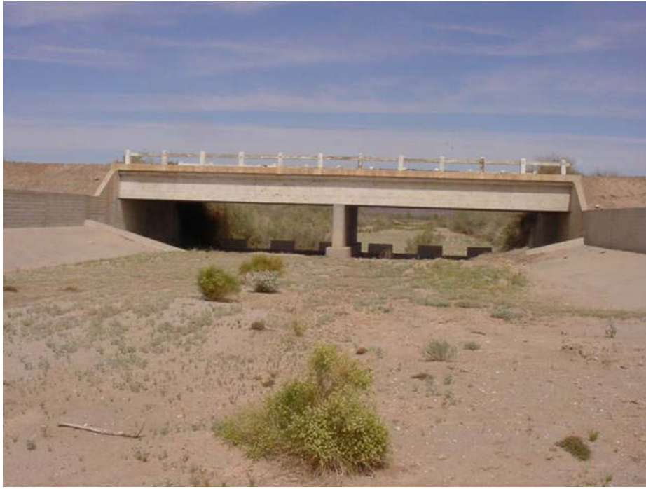
Photo 3: View of WUS-2 crossing looking north.
