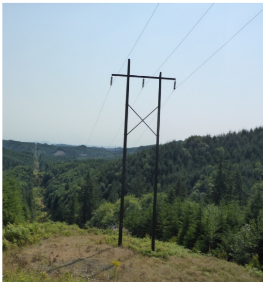
Figure 2-1. Existing Two-Pole Wood Structure
