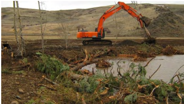
Figure 4. 300 series Track-mounted excavator
