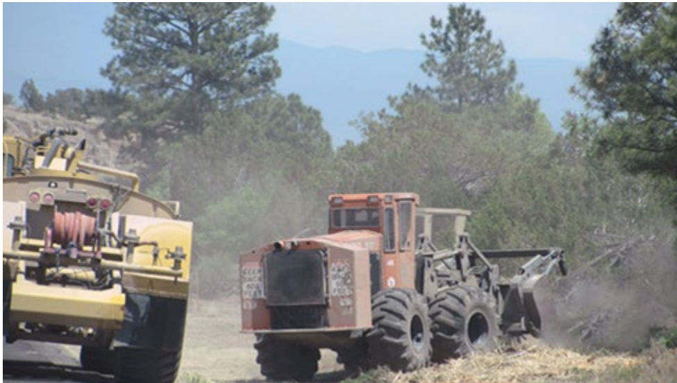
Figure 2-1: Masticators used to chip biomass in place
