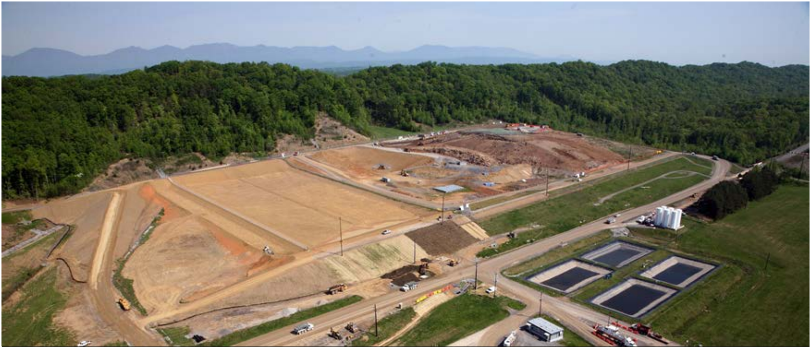
The current onsite disposal facility, the Environmental Management Waste Management Facility
