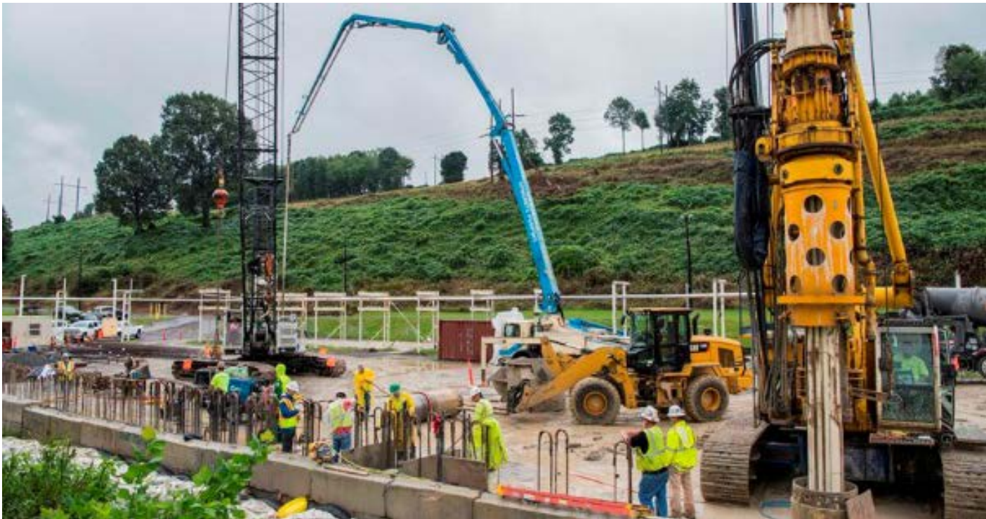
Crews constructing the retaining walls for the Mercury Treatment Facility
