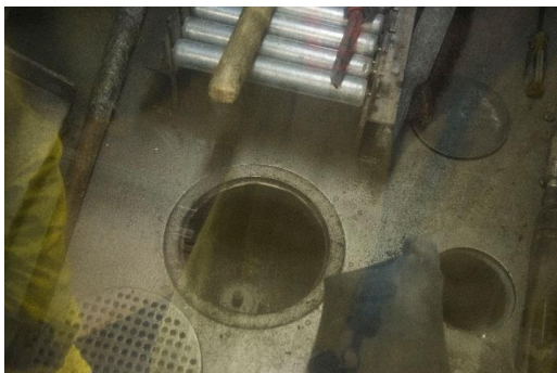
Figure 2. Floor of the Knockout Glovebox
