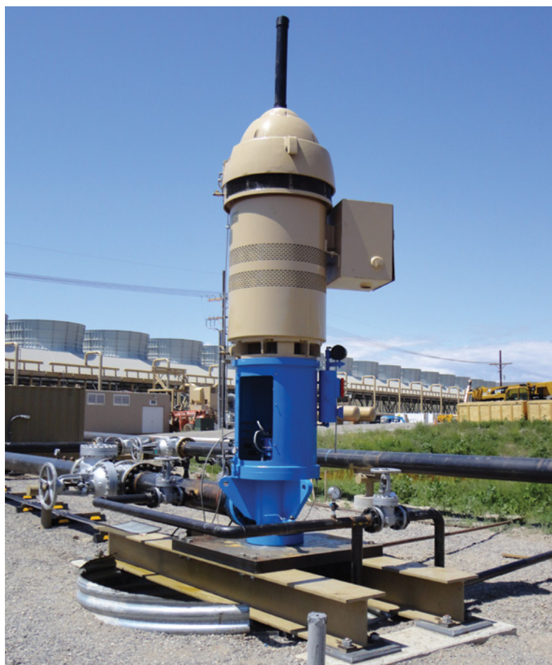
A submersible pump on a geothermal production well in western Oregon. Photo credit: Alan Ofsoski
