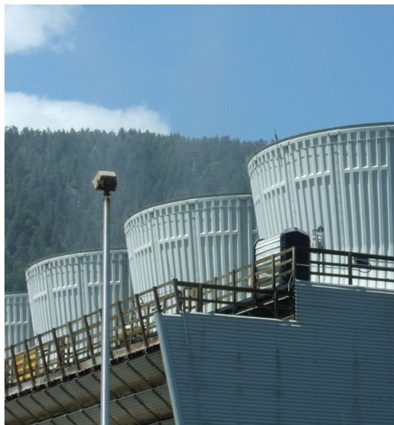
An evaporative cooling tower at Socrates Geothermal Power Plant (The Geysers, California). Photo credit: Geothermal Resources Council
