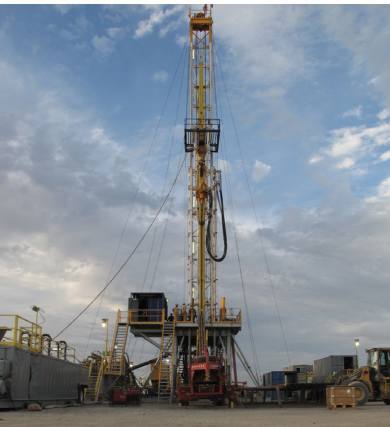
Drilling a 9,000-foot geothermal test hole in Fallon, Nevada. Photo credit: Andrew Tiedeman
