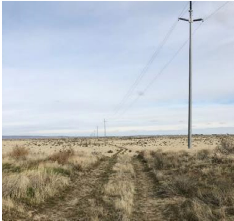
Figure 3-23. KOP-3 – White Bluffs – Single Pole Steel Structures Near Access Road Facing North
