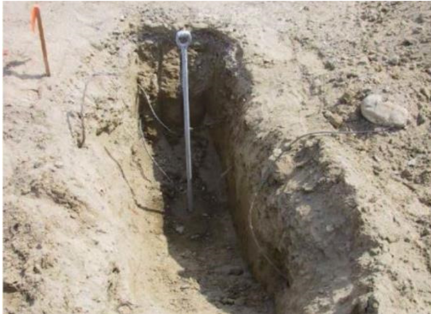
Figure 2-6. Plate Anchor Hole and Anchor Rod
