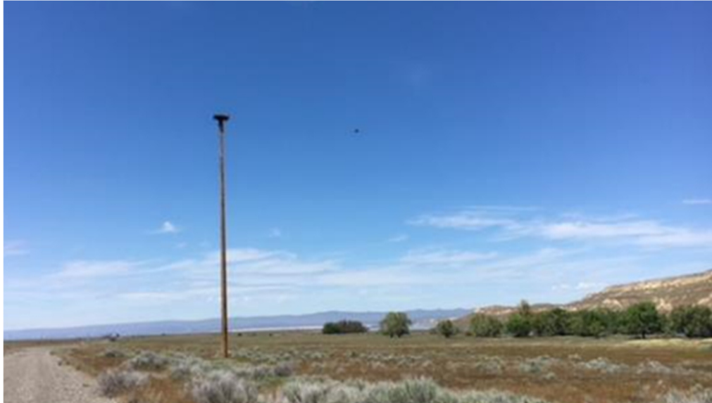
Figure 3-2. Osprey Nesting Platform near Pole Structure 24/6
