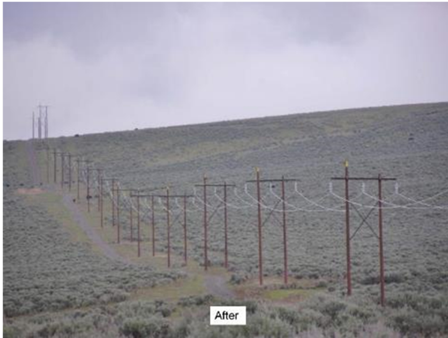
Figure 3-26. Structures and Access Roads on Rebuilt Section North of Project (After)
