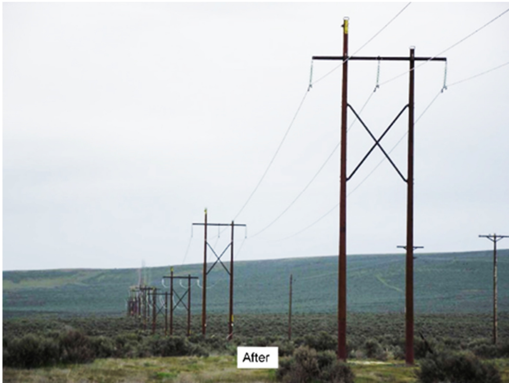
Figure 2-2. Completed Transmission Line Rebuild North of Project Limits (After)
