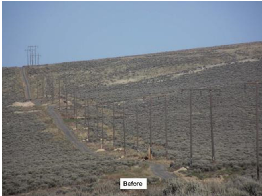
Figure 3-25. Structures and Access Roads on Rebuilt Section North of Project (Before)
