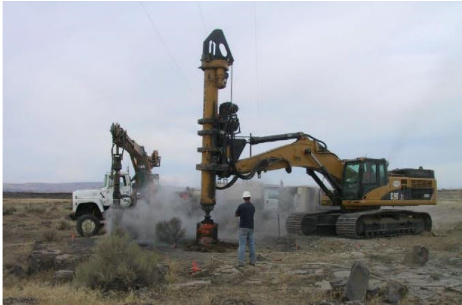
Figure 2-5. Pole Hole Excavation
