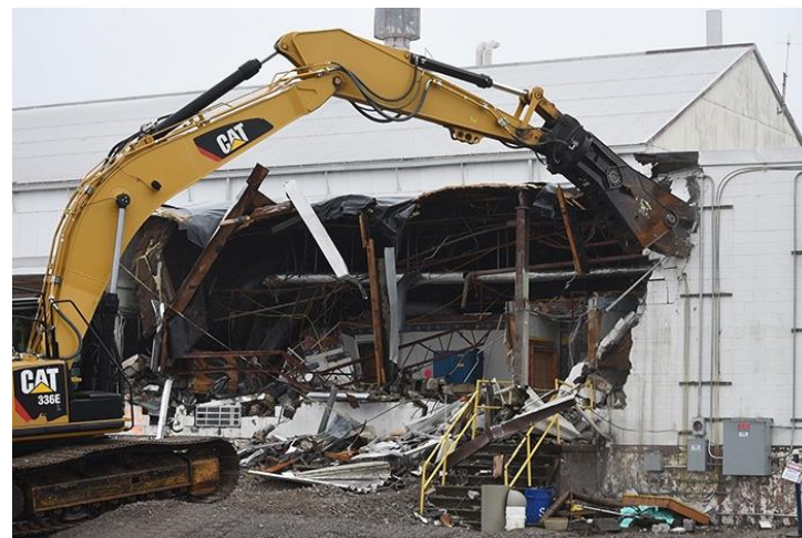
Oak Ridge - Demolish Building K-1037 scheduled for completion later this year
