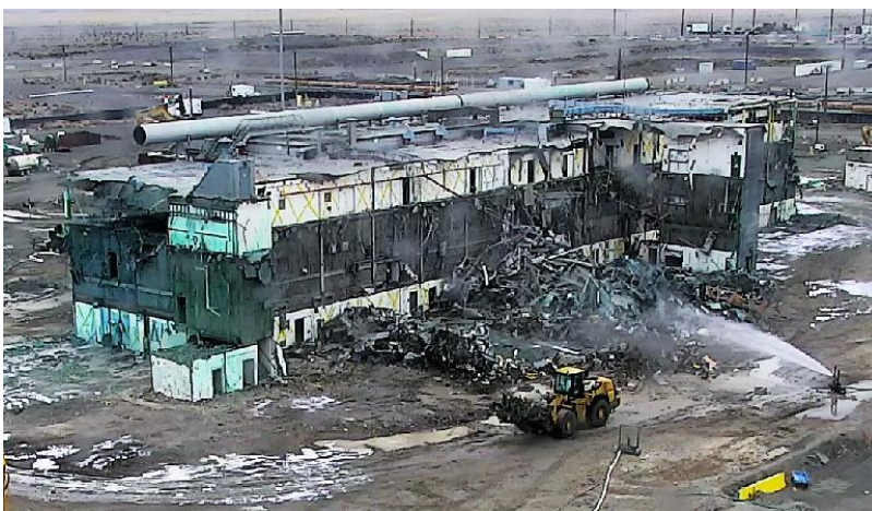
Richland - Complete demolition of the Plutonium Finishing Plant
