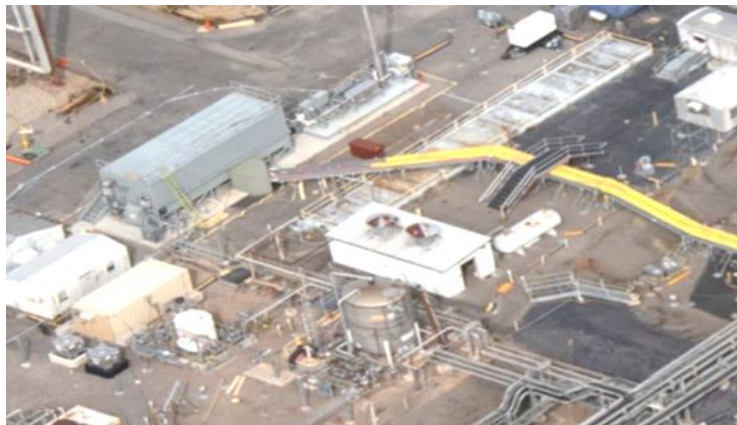
Savannah River - Tank Closure Cesium Removal treatment unit operation
