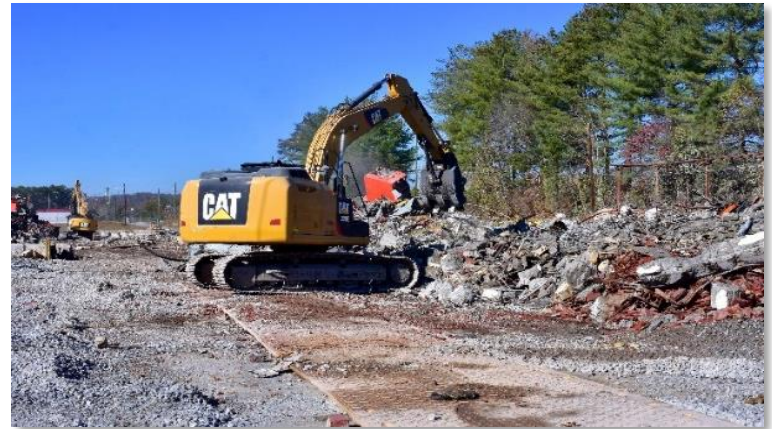
Demolition of East Tennessee Technology Park facilities
