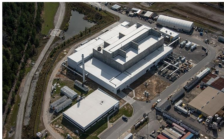
Salt Waste Processing Facility
