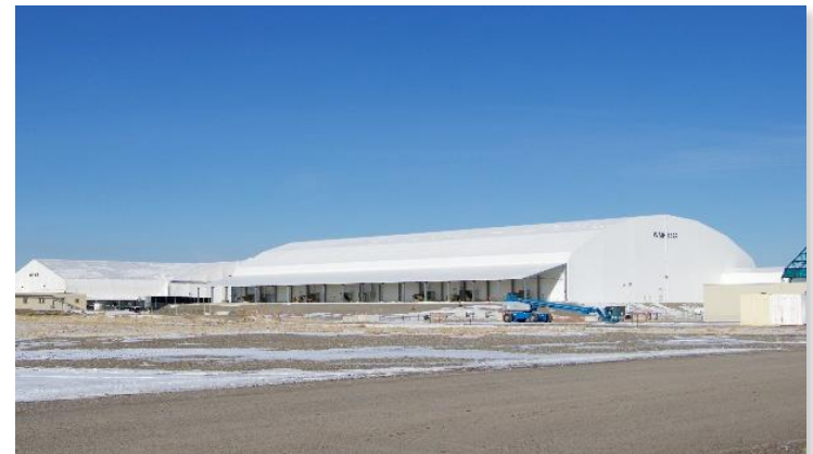
Accelerated Retrieval Project Enclosure 9
