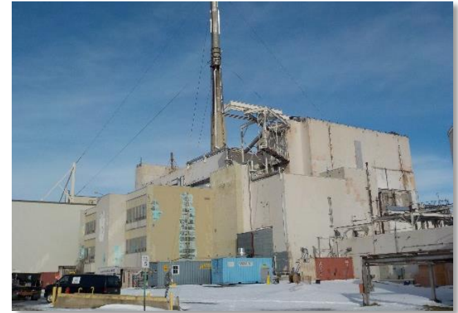
Main Plant Process Building at West Valley
