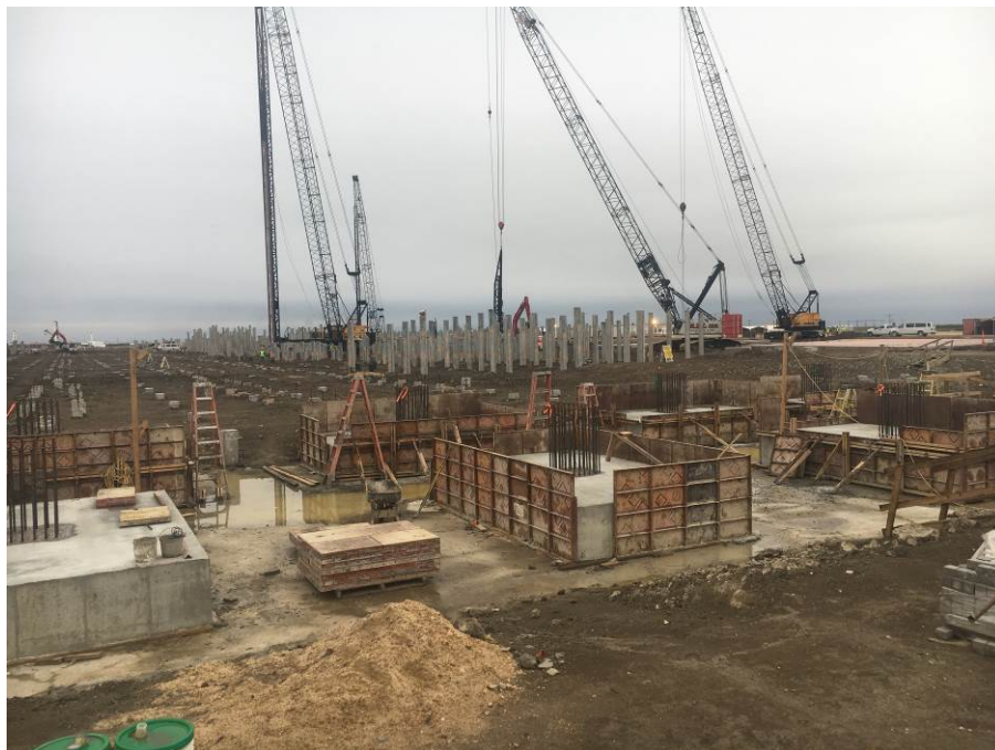
Train 6 – Last Pile Caps Concrete
