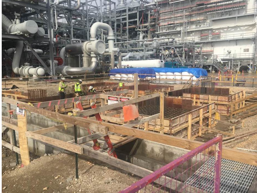
Train 6 – R10 Pipe Rack Pile Caps formwork in progress
