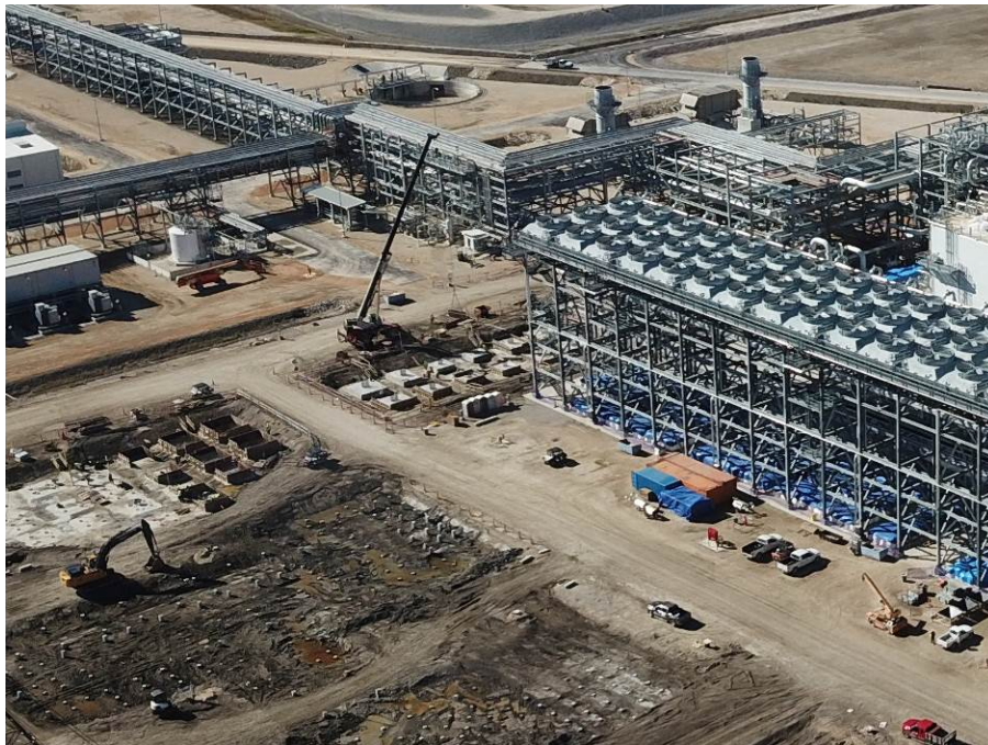
Train 6 – R10 Pipe Rack Progress
