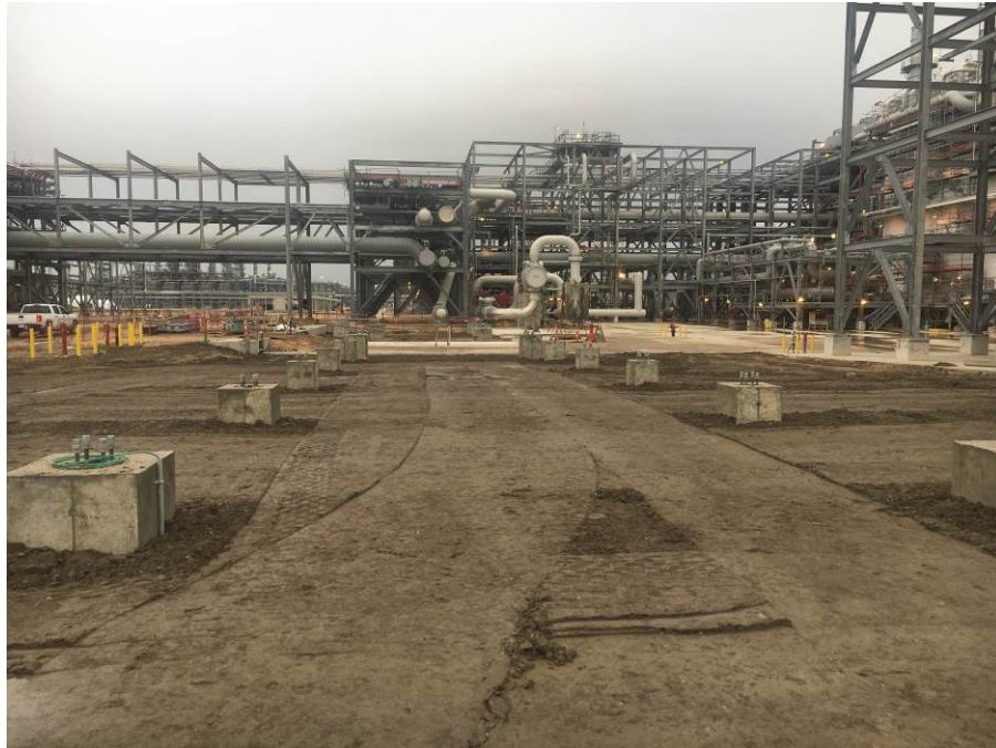
Train 6 – R10 Pipe Rack Pile Caps and Pedestals Complete
