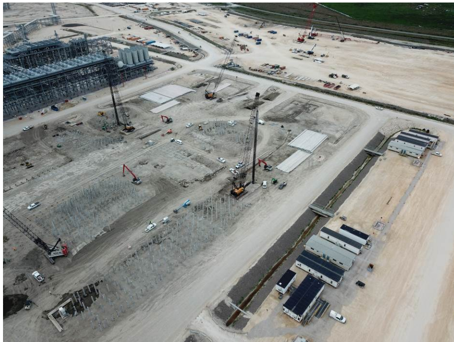
Train 6 – Aerial View of Piling Progress and Support Facilities
