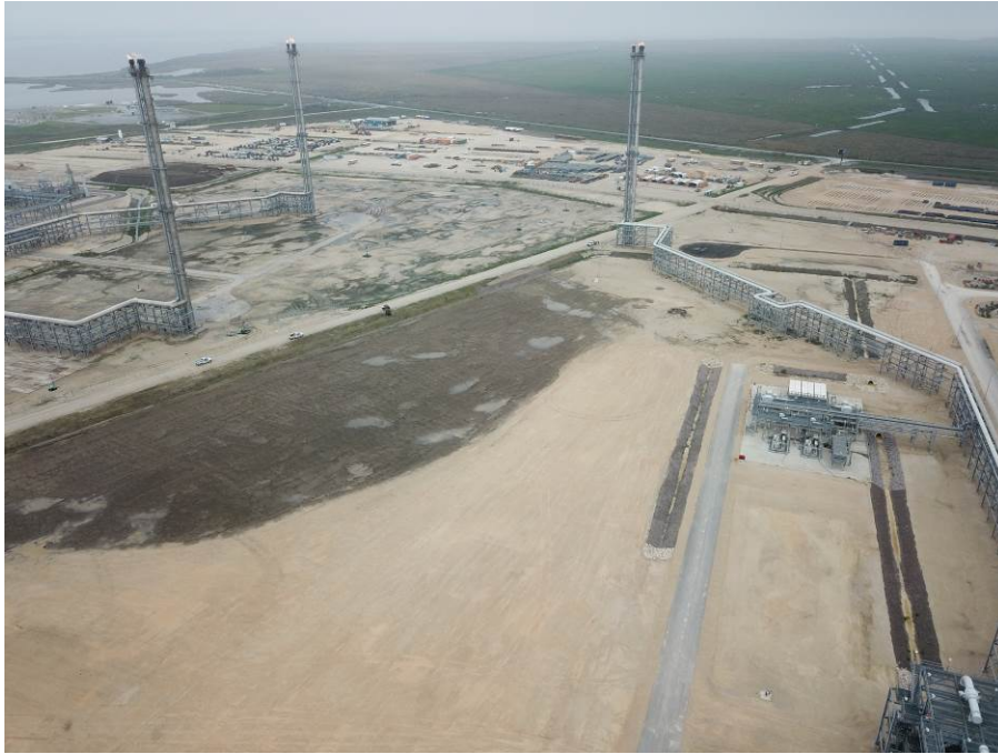
Train 5 – Flare Area Grading
