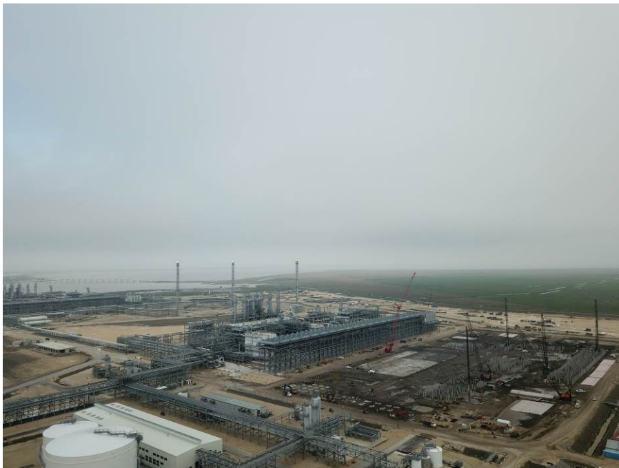
Trains 5 & 6 – Aerial View
