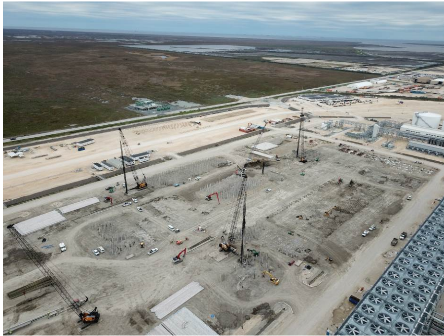
Train 6 – Aerial View showing Piling and R10 Pipe Rack Progress
