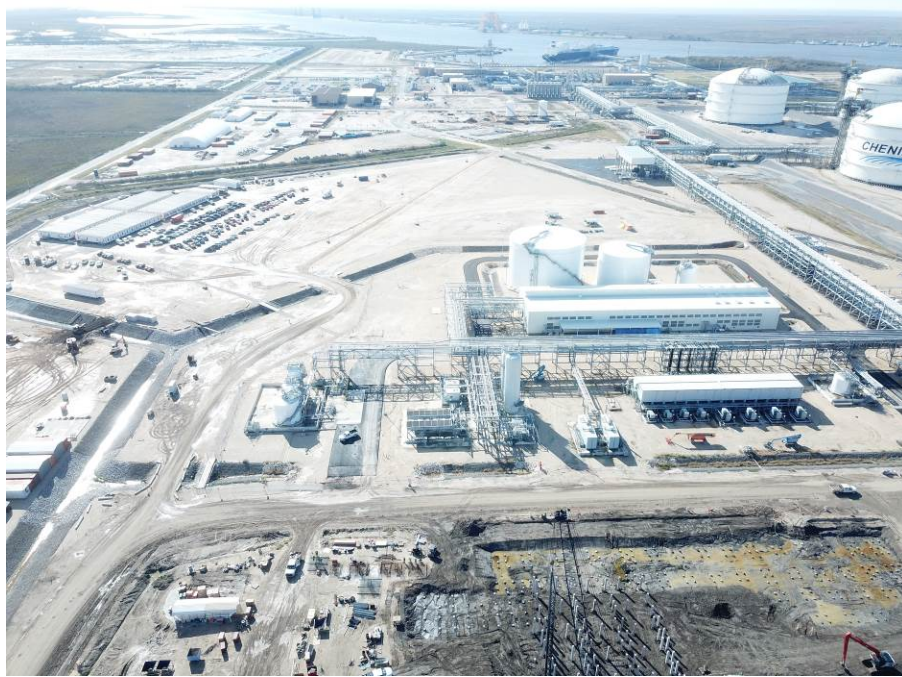
OSBL – Utility Area Asphalt Paving Complete
