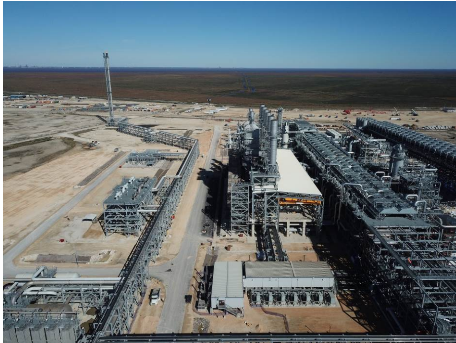
Train 5 – Asphalt Paving Complete
