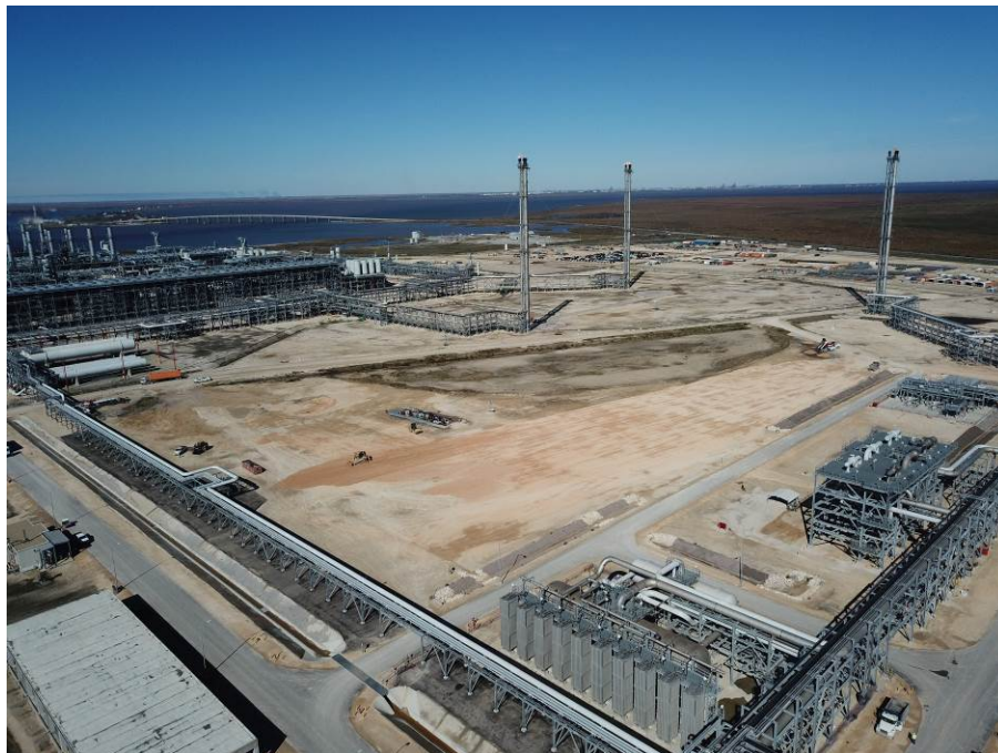
Train 5 – Flare Area Grading
