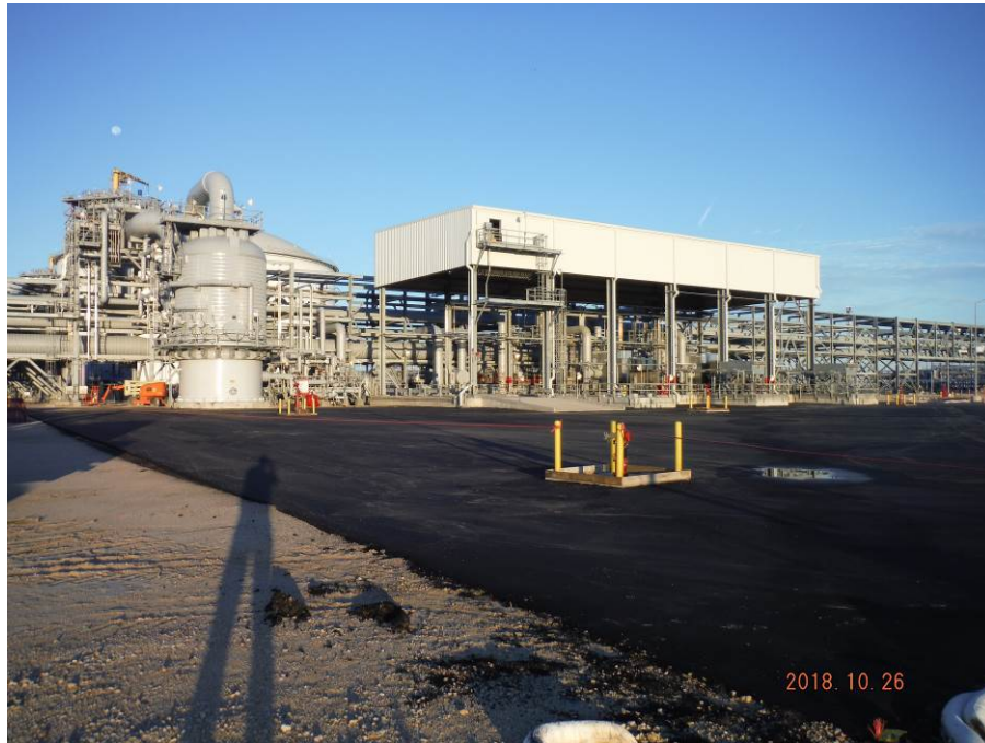
OSBL – Asphalt Paving Progress in BOG Area
