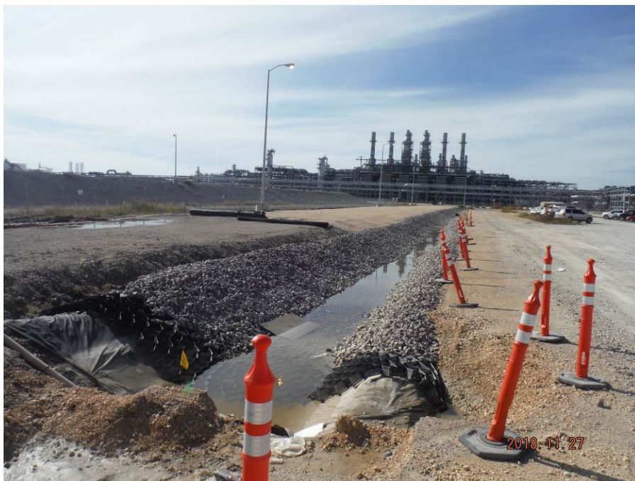
Stage 3 CMT Complex Road and Drainage Ditch
