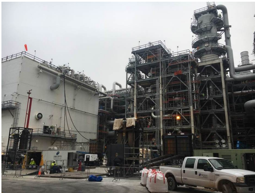
Train 5 – Perlite Loading in Progress
