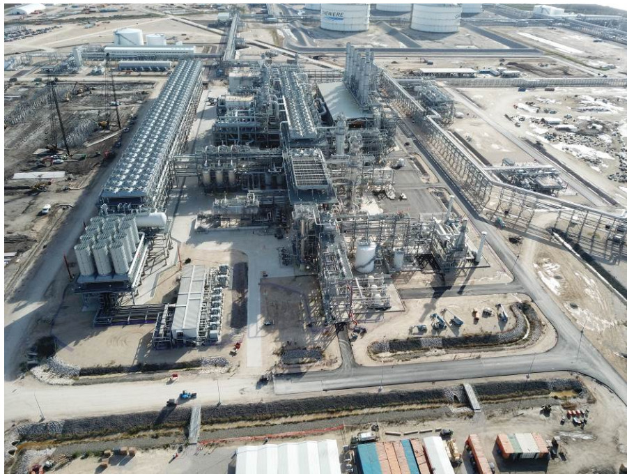
Train 5 – Aerial View
