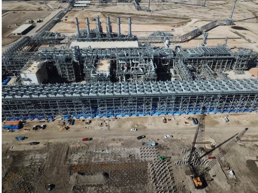
Train 5 – Aerial View
