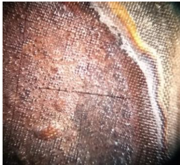
Delamination of bipolar membrane at elevated temperatures.
