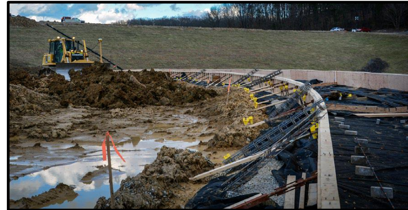
Another view of the spillway during construction.
