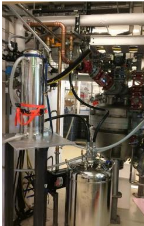
Custom vacuum system for Andritz pretreatment & extraction vessel
