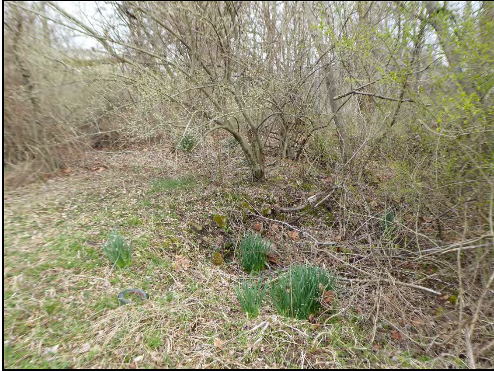
Figure 29: Site area facing southwest. Note south foundation wall in center of photograph.
