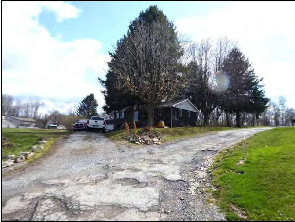
Photo 13: 3721 Collins Ferry Road, northwest (rear) and southwest (side) façades, facing northeast.
