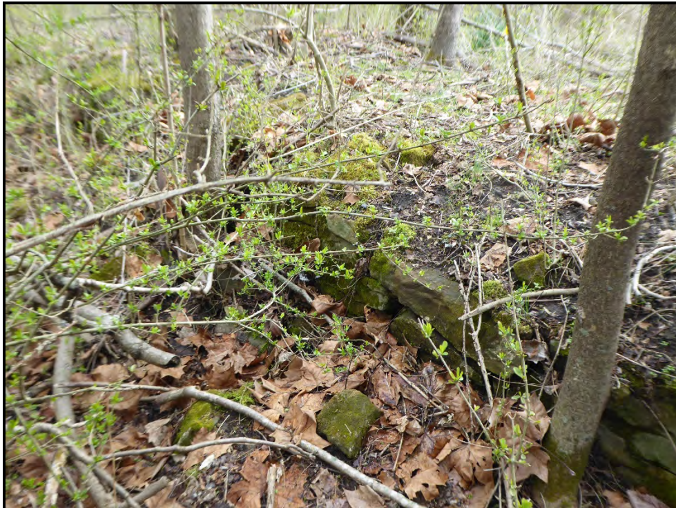
Figure 34: East foundation wall, facing north.
