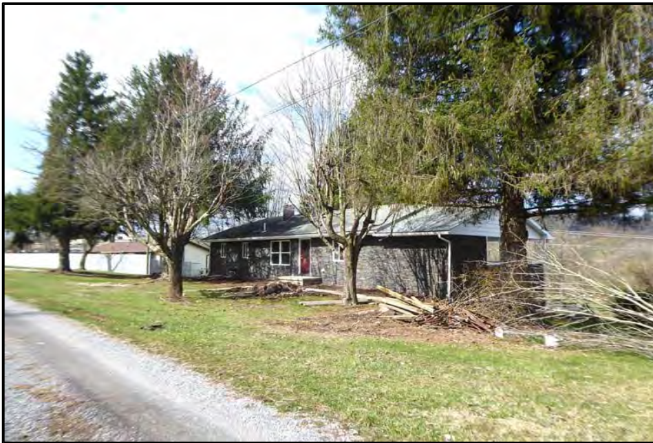
Photo 12: 3721 Collins Ferry Road, southeast (front) and northeast (side) façades, facing southwest.
