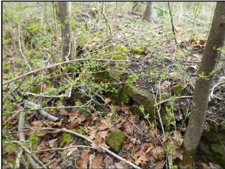
East foundation wall, facing north.
