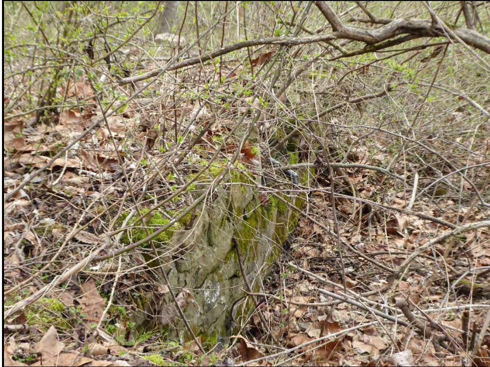
Figure 35: South foundation wall, facing southwest.
