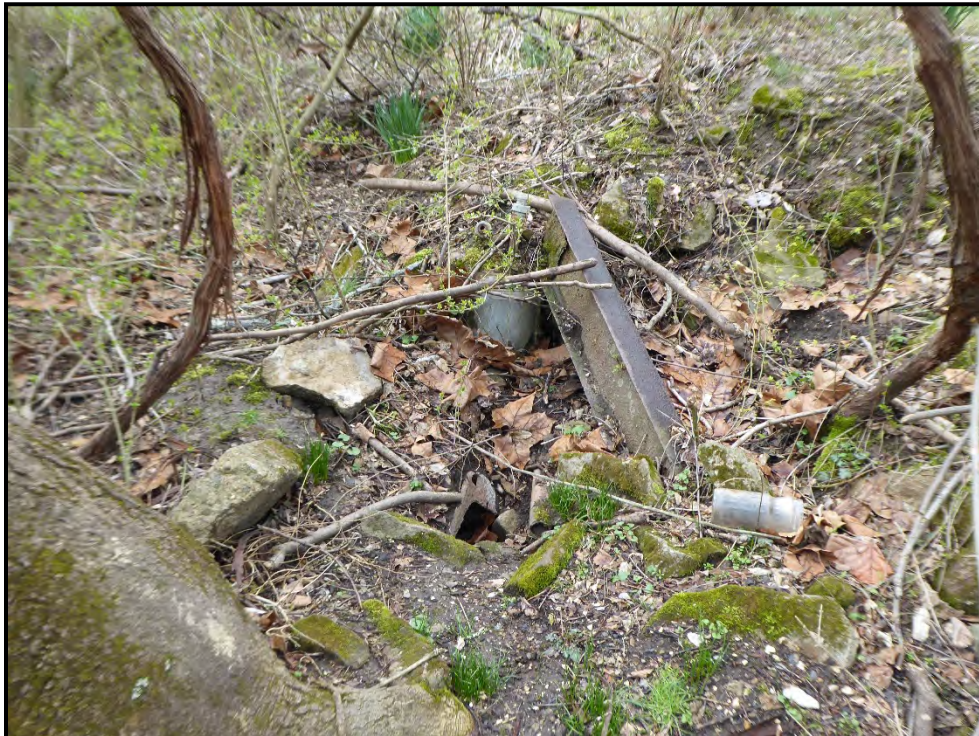
Figure 38: Rubble within the foundation.
