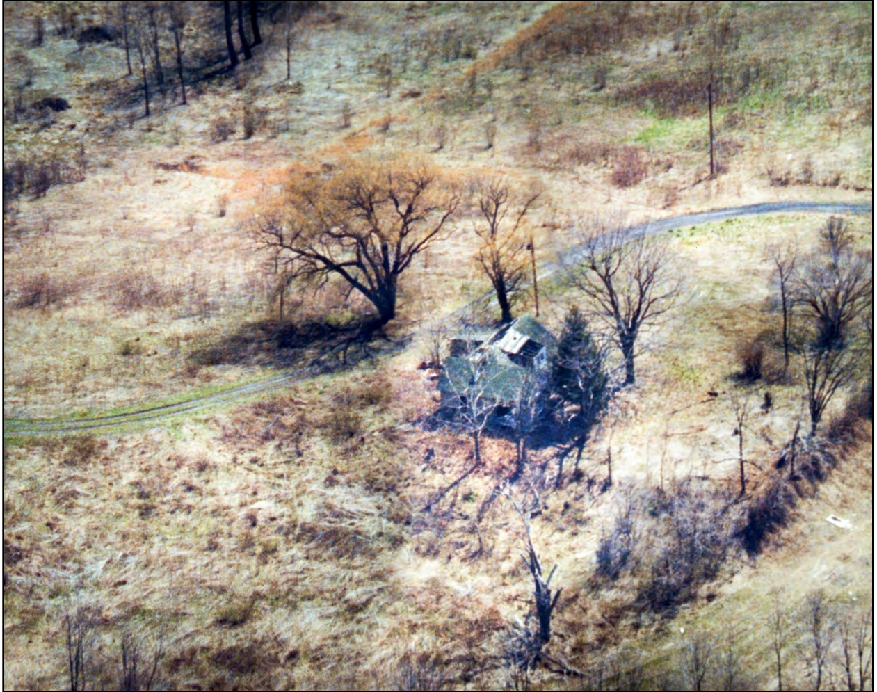
Figure 12: Aerial photograph of the house taken shortly before its demolition, ca. 1980, facing southeast (courtesy NETL).
