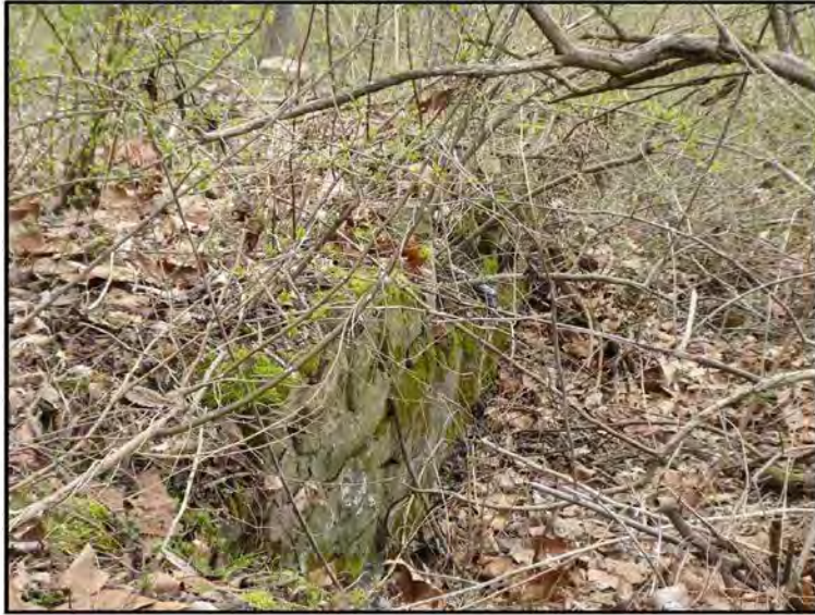
South foundation wall, facing southwest.
