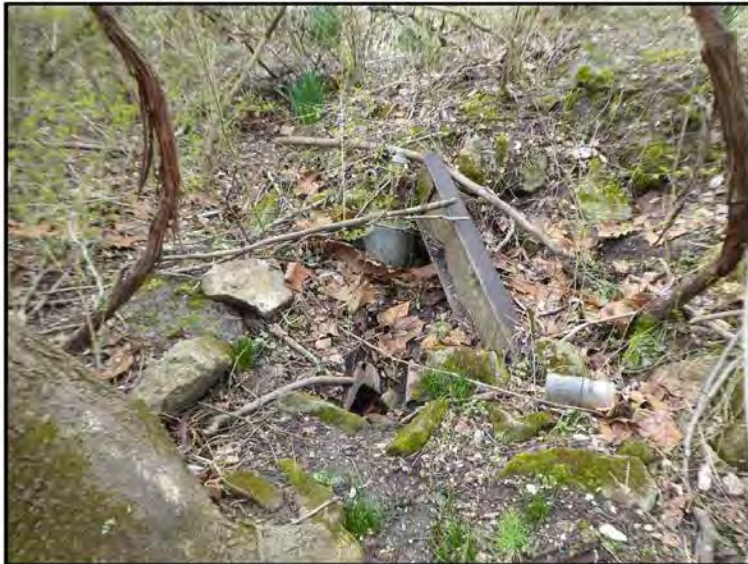
Rubble within the foundation.
