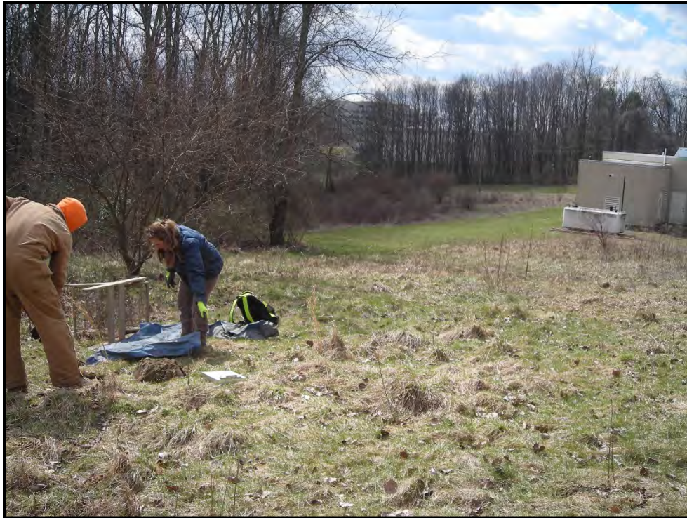
Figure 49: Excavation of the STP at the reported location of the concrete features, facing southwest.
