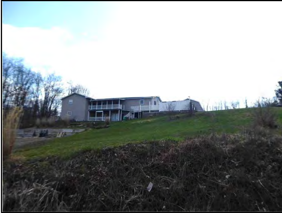
Photo 15: 3734 Collins Ferry Road, northwest (rear) and southwest (side) façades, facing northeast.
