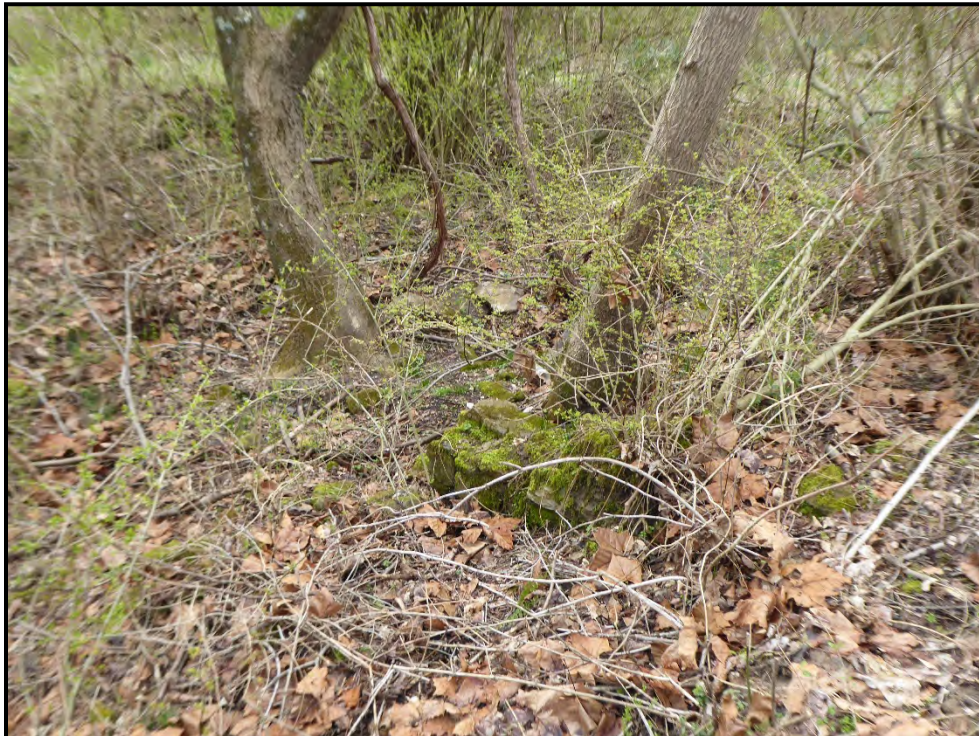
Figure 36: West foundation wall, facing south. Note interior portion of foundation in center of photograph.
