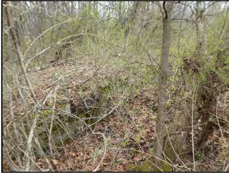
North foundation wall, facing northeast.
