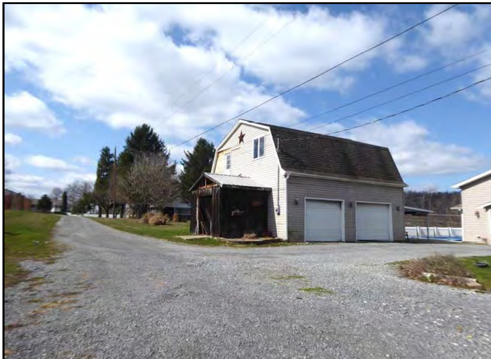
Photo 16: Garage at 3734 Collins Ferry Drive, southeast (side) and northeast (front) façades, facing southwest.
