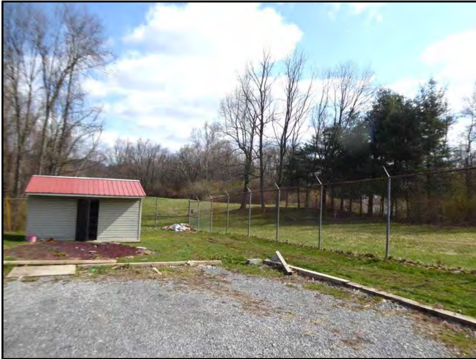
Photo 10: View at northeast terminus of Farrell Street at 3437 Collins Ferry Road, facing east towards site of proposed renovations to Building 42.
