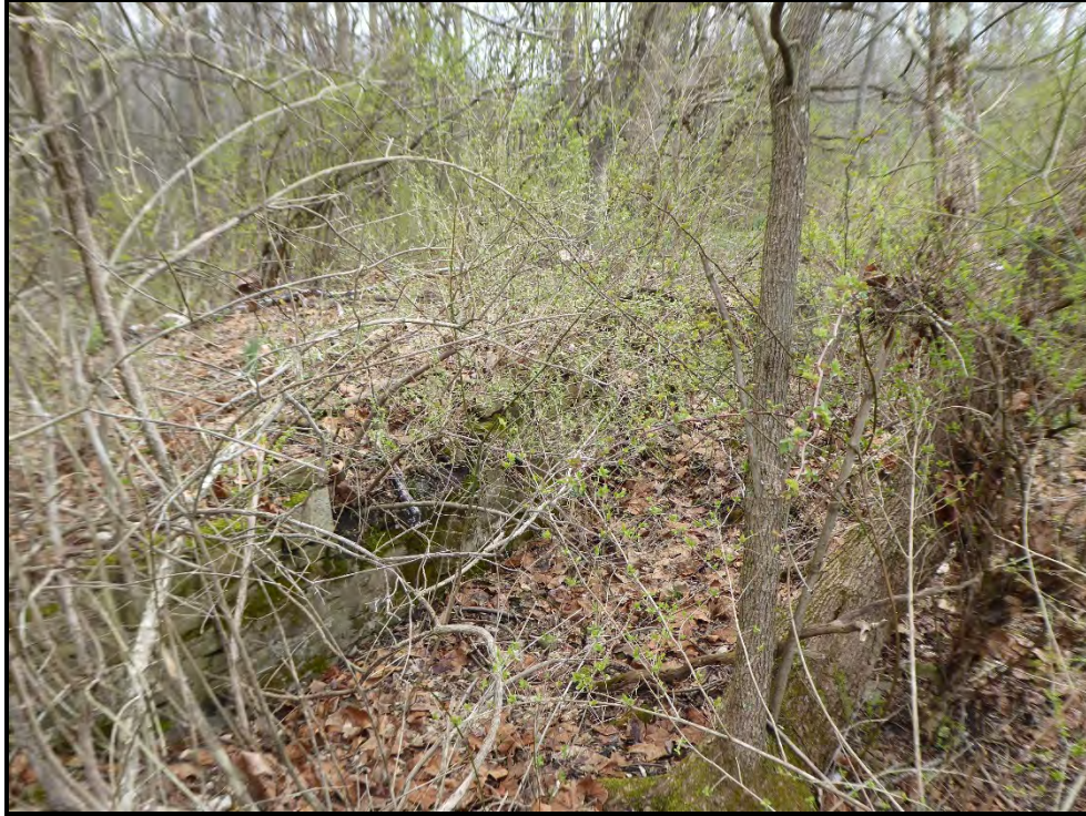
Figure 33: North foundation wall, facing northeast.
