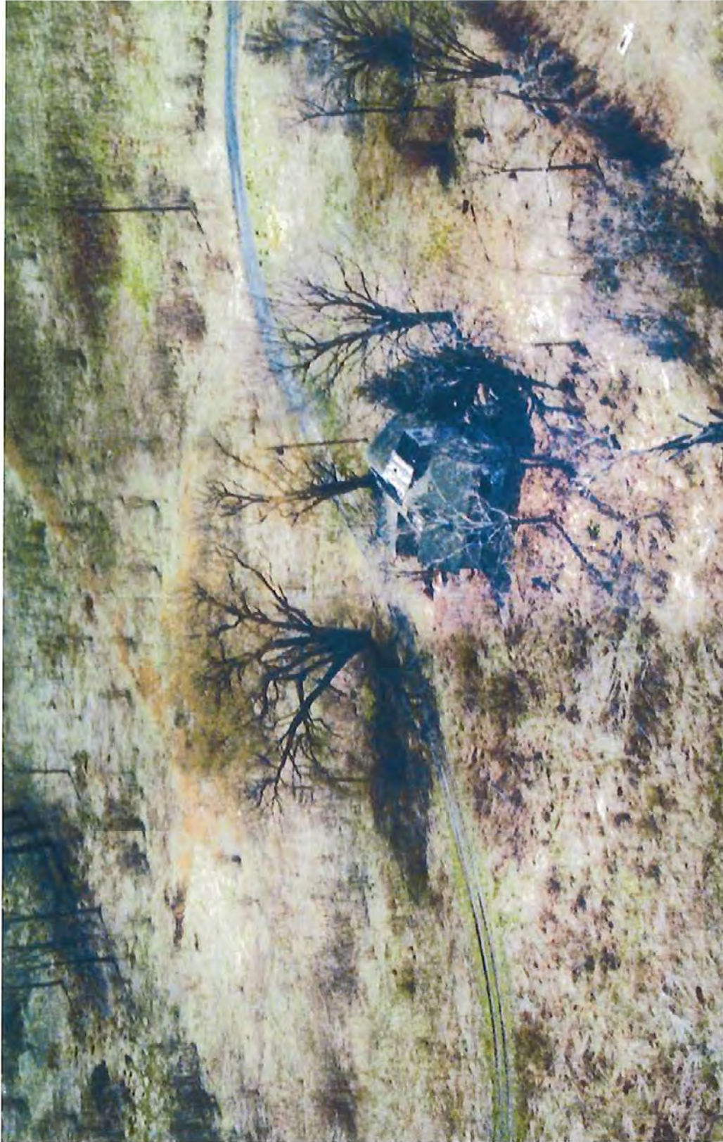
SINCLAIR HOUSE AERIAL SHOT. CAMERA FACING NORTHWEST. THE HOUSE WAS TORN DOWN BY THE NAVY/DOE AFTER ACQUISITION IN 1980. DATE RANGE ON THE PHOTO WOULD BE BETWEEN 1978 AND 1980.
