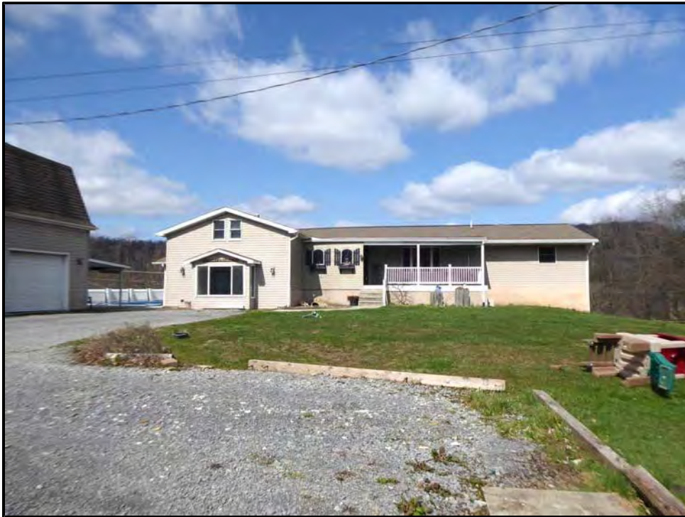
Photo 14: 3734 Collins Ferry Road, southeast (front) façade, facing northwest.
