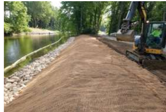
Bank stabilization, South River, Virginia
