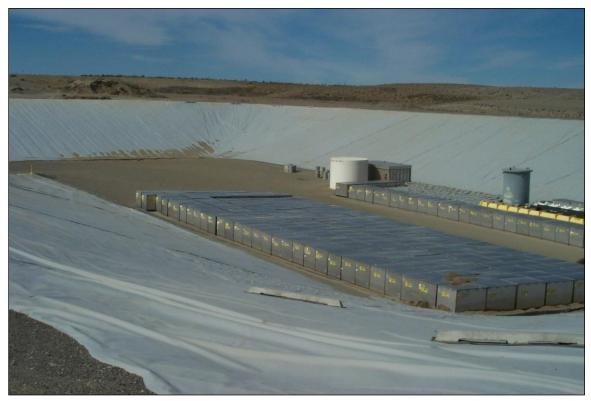
Figure 2–22. Lined Disposal Trench in Low-Level Radioactive Waste Burial Ground 218-W-5
