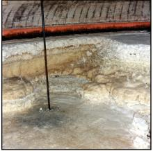
Figure 2–9. Crystallized Salt Cake Inside One of the Hanford Site's Waste Tanks
