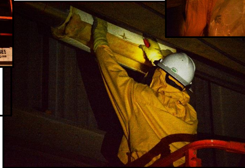
Once cut, sections of fiberglass insulation are quickly removed.
