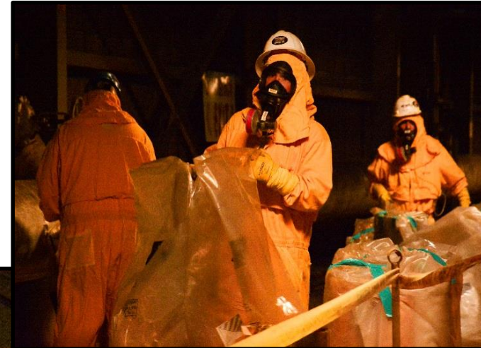
Project workers bag some of the fiberglass insulation for disposal.
