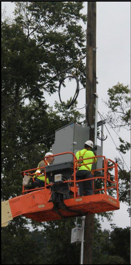
← Workers at the X-6609 install one of the VFD panels
