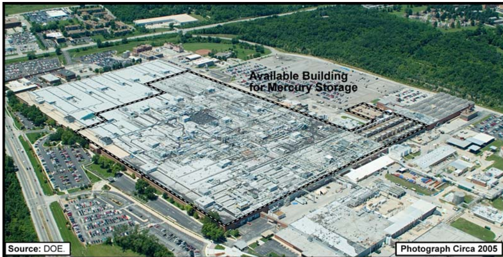
Existing Main Manufacturing Building at the Kansas City Plant
