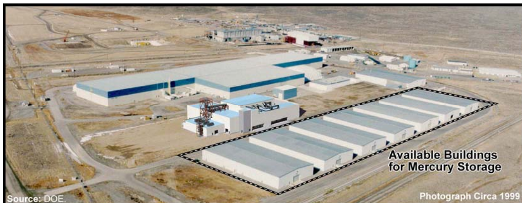
Existing Storage Buildings at the Radioactive Waste Management Complex at Idaho National Laboratory
