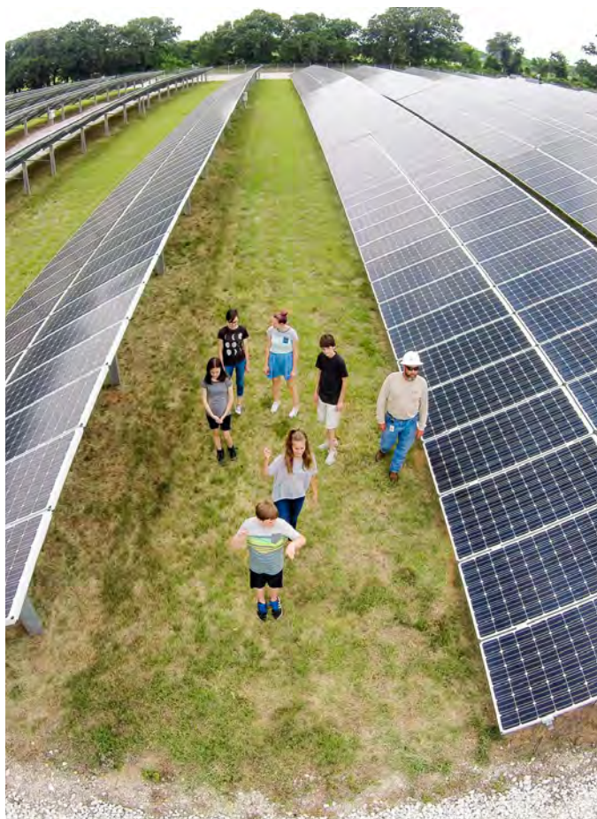
Students visit the 2-megawatt CoServ Solar Station in Krugerville, Texas.
