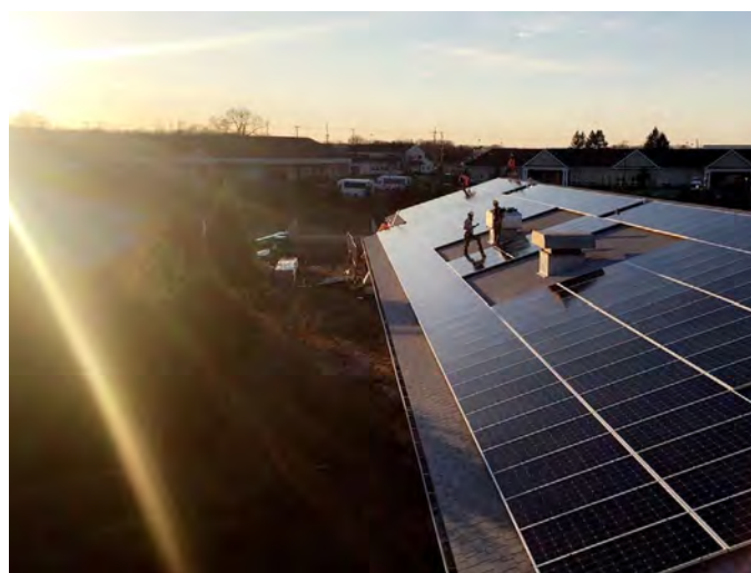
Gorgeous evening on a solar array installation in Delran, New Jersey.
