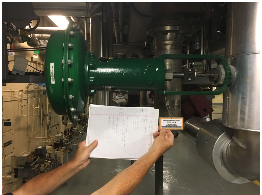
Figure 1: Steam Isolation Valve
