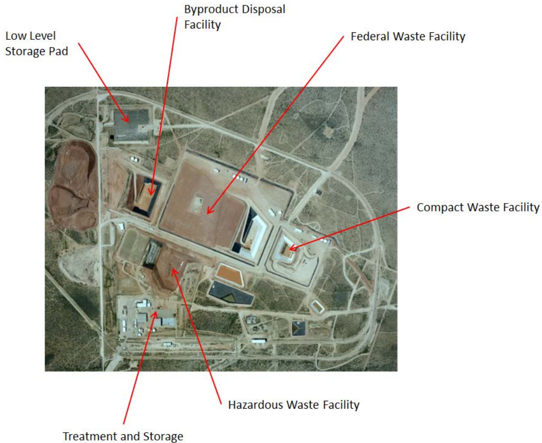
Figure 3-8 Waste Control Specialists LLC Waste Management Facilities (Source: WCS 2016d)
